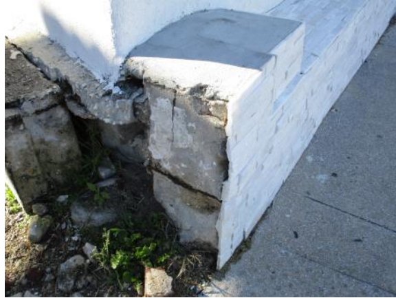
End of wall facing Bravo Lane
