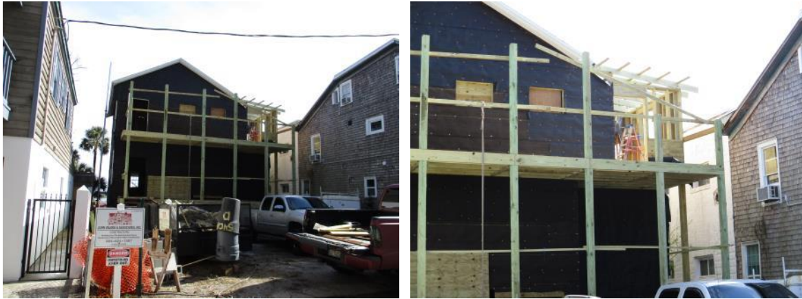
Rear, or western, façade facing Marine Street
