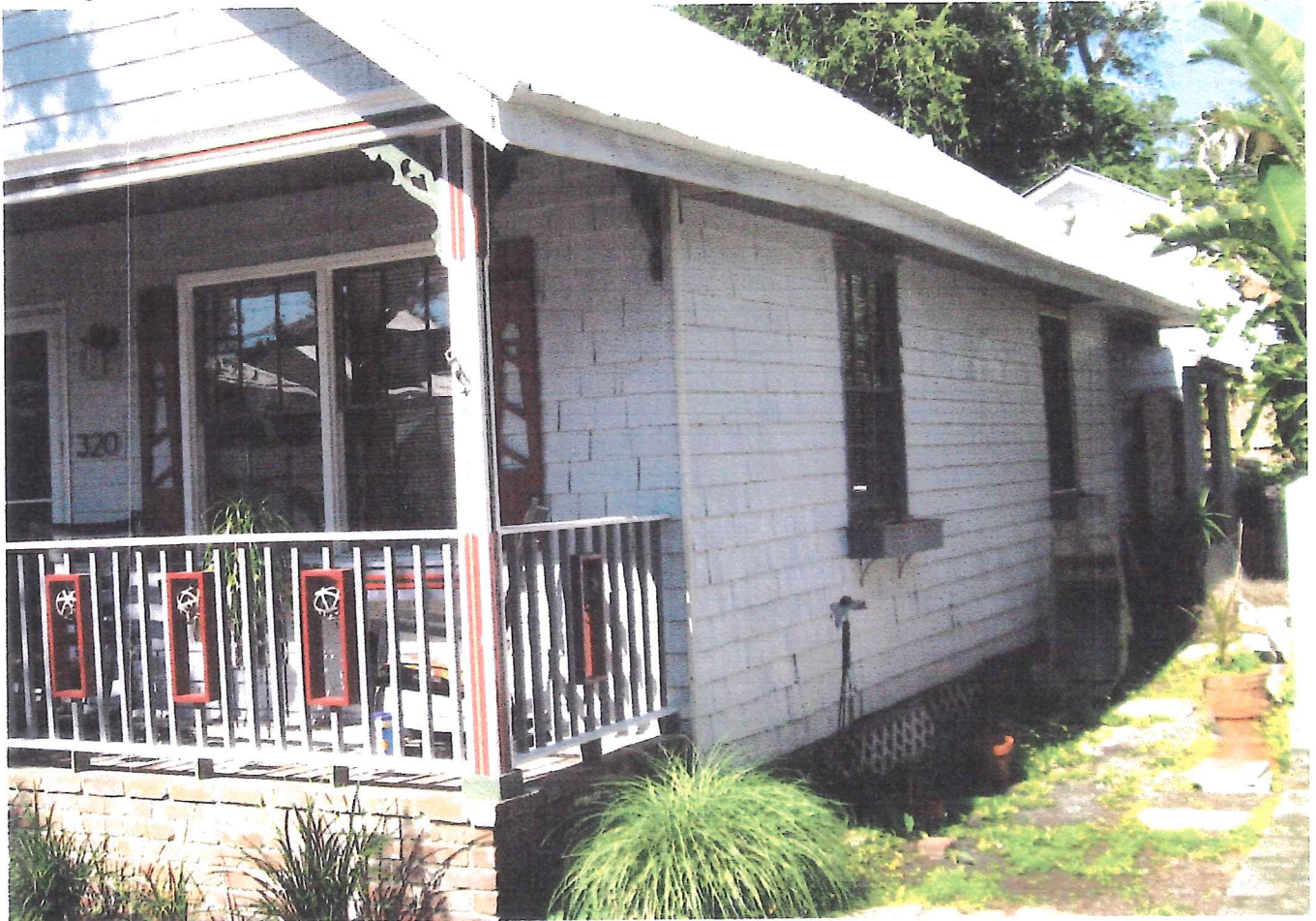
EXISTING NORTH FACADE
