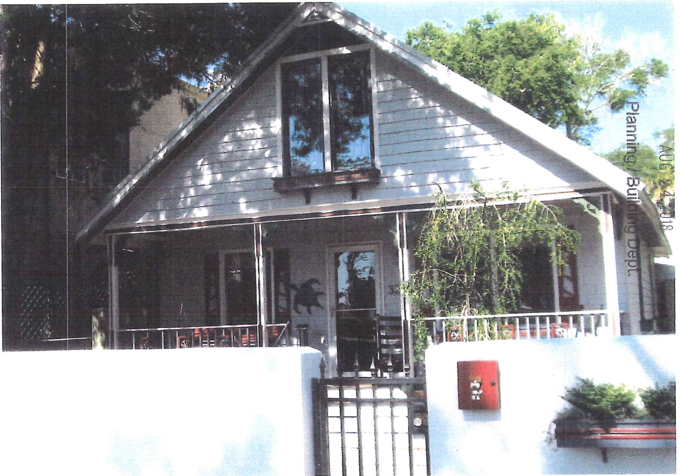
EXISTING EAST FACADE
