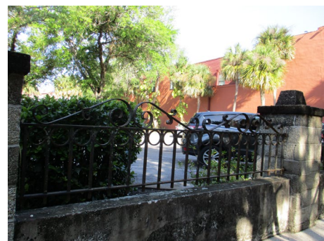
The Existing Wrought Iron Work
