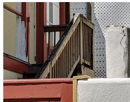
Existing Staircase and Porch
