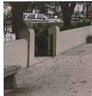
CATHEDRAL WALL EXISTING COLOR OR BUILDING ACROSS ST. GEORGE STREET
