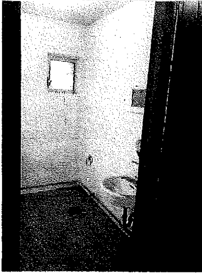
Interior – Second Floor Bathroom #1
