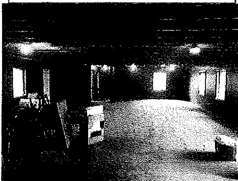
Interior – Second Floor- West side
