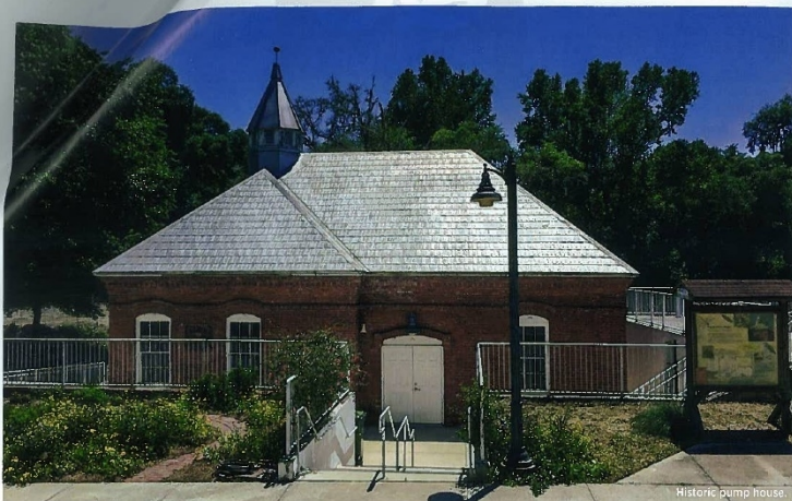
Historic pump house
