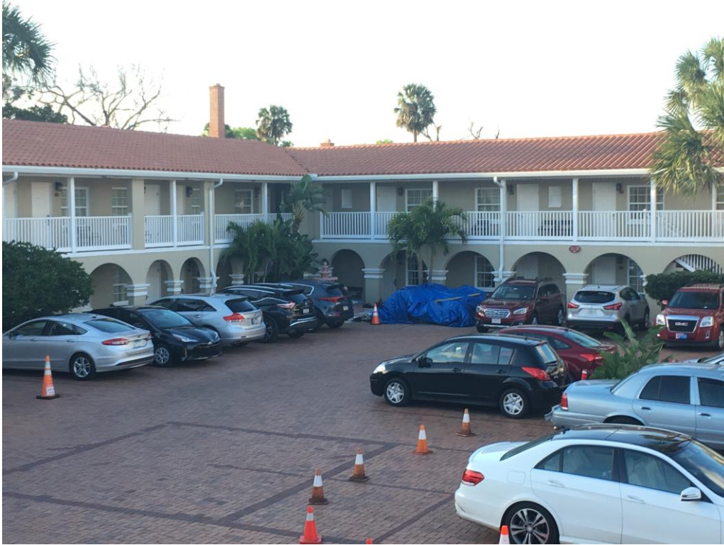
New Construction – Photo 11.5 Corner area where fountain will be removed and elevator shaft and stair will be constructed.
