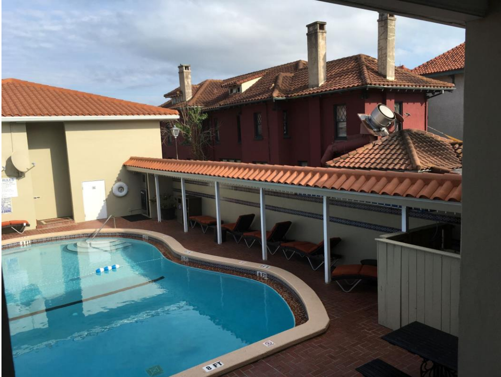
Roofs and Roofing – Photo 1.2 View of existing roofing
