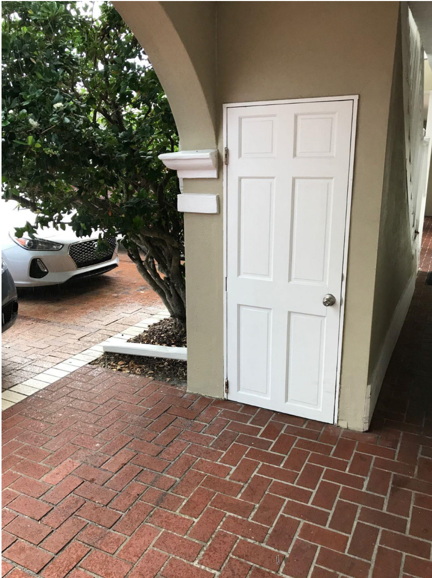
Exterior Doors – Photo 5.1 Typical exterior 6-panel door under stair
