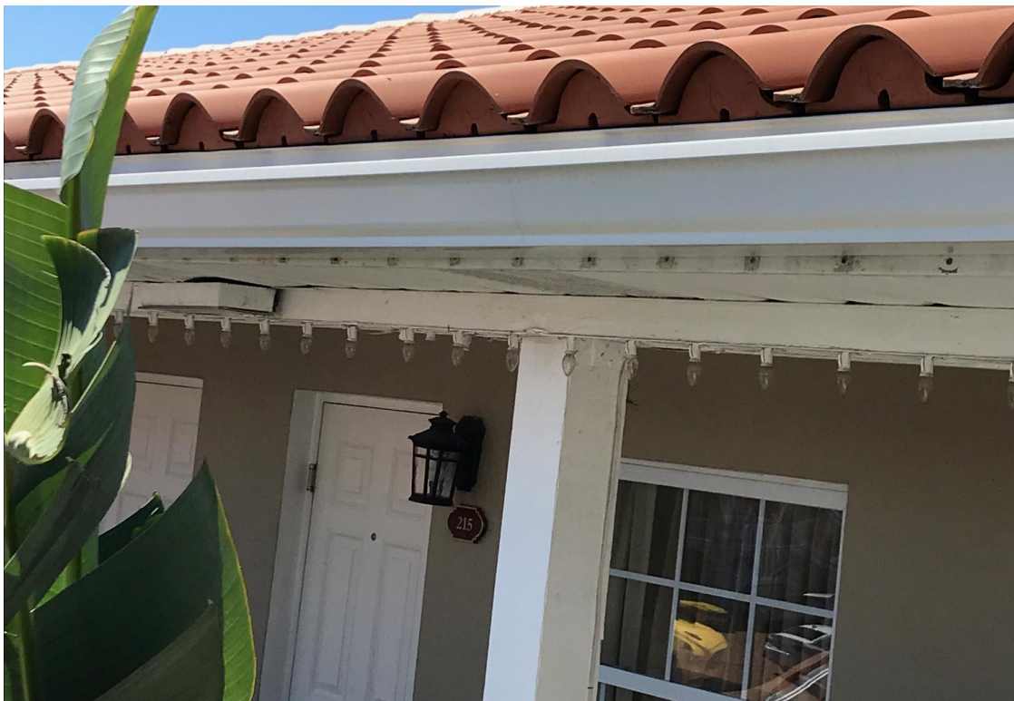
Exterior Electrical/Mechanical – Photo 8.2 Existing lighting fixture
