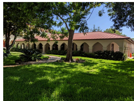
Exterior of Building
