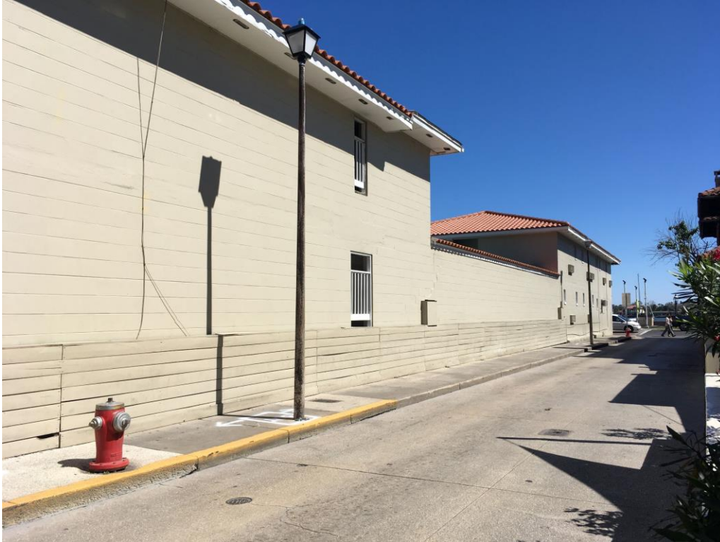
Exterior Finishes – Photo 2.1 View on Hypolita. Exposed painted CMU and wood “fence”
