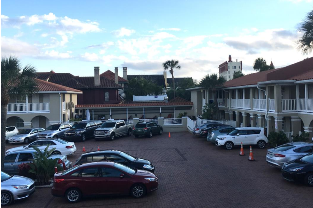
New Construction – Photo 11.1 Pool area where walkway connecting the second floors will be constructed – viewed from parking.
