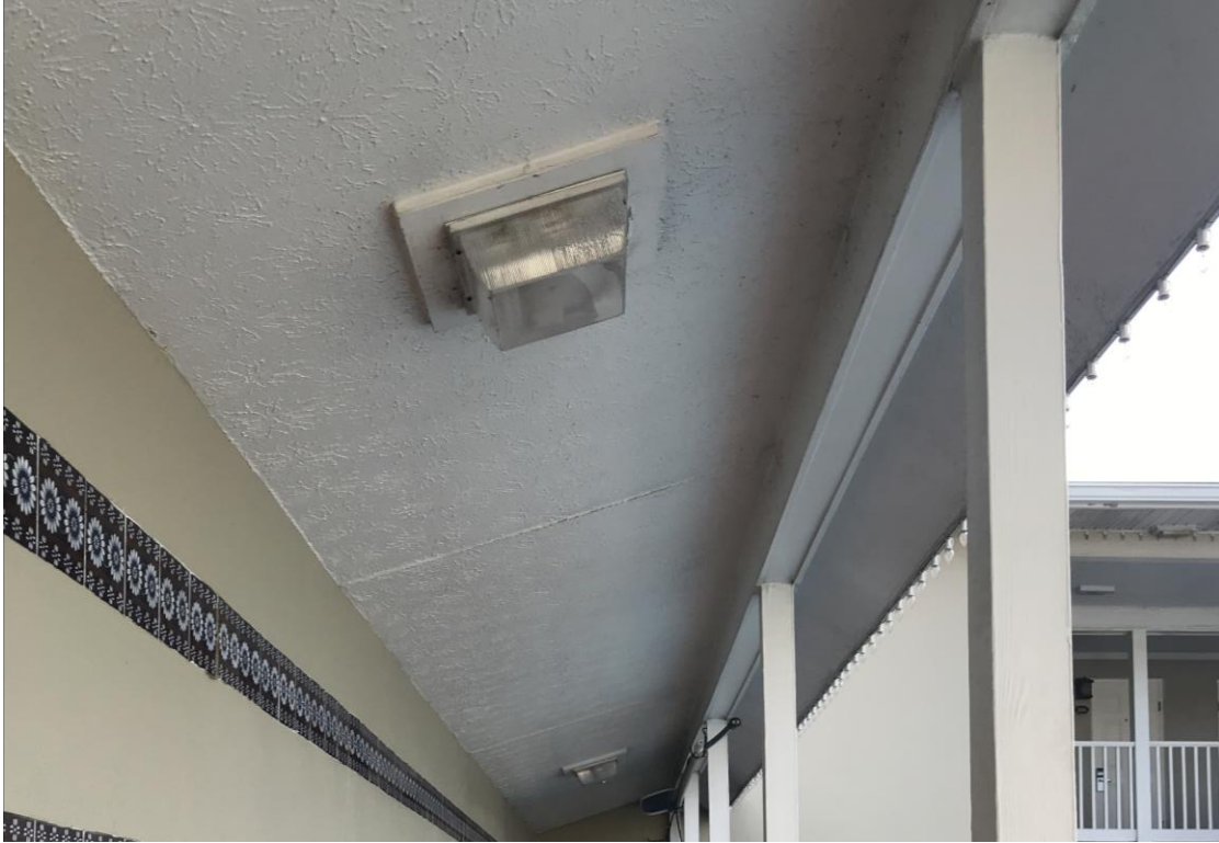
Exterior Electrical/Mechanical – Photo 8.1 Existing lighting fixture
