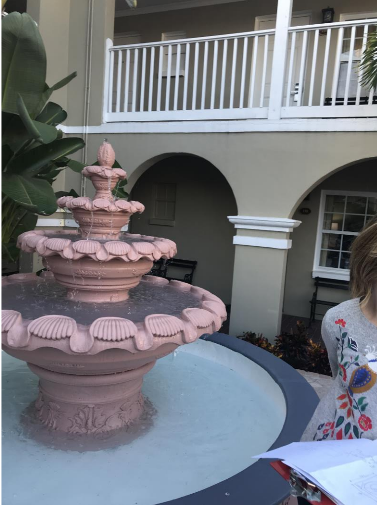
Parking, Landscape, or other site feature – Photo 10.1 Fountain to be removed
