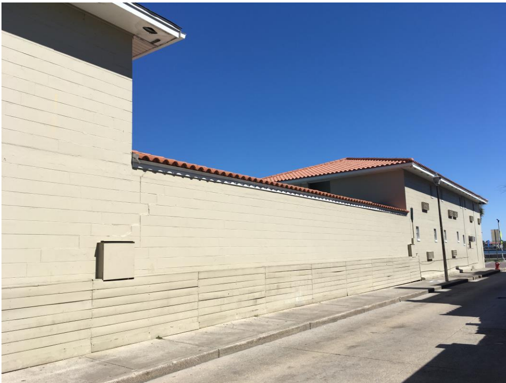
New Construction – Photo 11.2 Pool area where walkway connecting the second floors will be constructed viewed from Hypolita Street.
