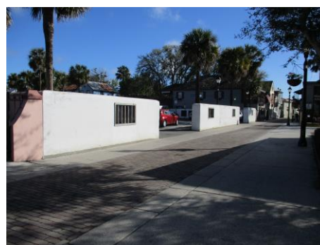
Street Facing Side of Wall
