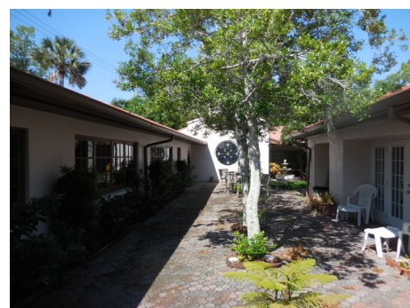
Existing Courtyard Area
