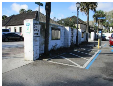
Parking Lot Side of Wall
