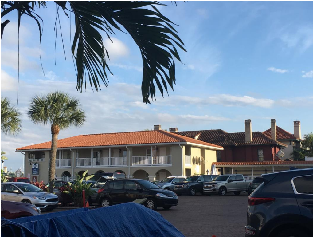
Roofs and Roofing – Photo 1.1 View of existing roofing
