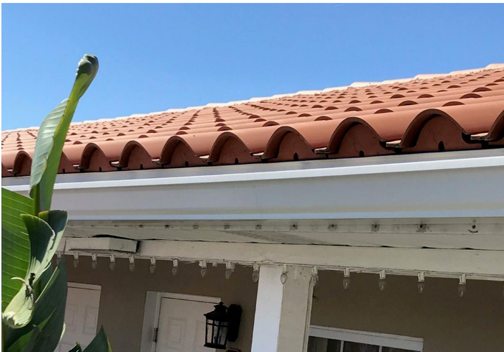
Roofs and Roofing – Photo 1.3 Close up view of existing roofing
