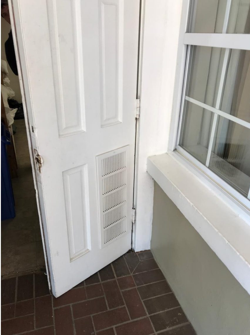
Exterior Doors – Photo 5.2 Typical exterior 6-panel door
