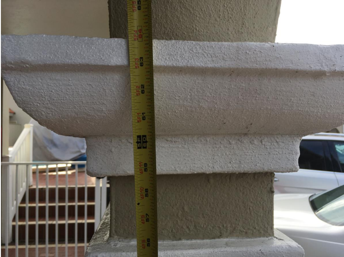
Exterior Finishes – Photos 2.3 Detail of typical finished façade of painted stucco
