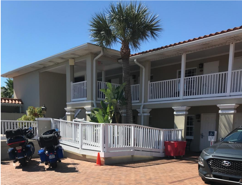
New Construction – Photo 11.3 Pool area where handicapped ramp will be removed and elevator shaft will be constructed.
