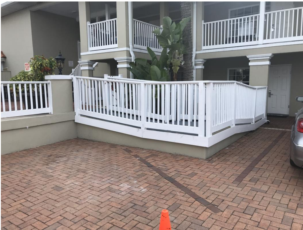
New Construction – Photo 11.4 Pool area where handicapped ramp will be removed and elevator shaft will be constructed – close up.
