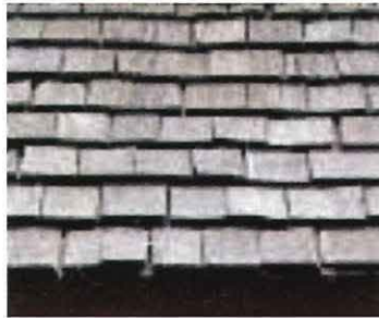
Wood shingle roof
