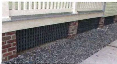
A new brick pier foundation matches historic materials and scale
