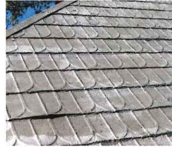
Stamped metal shingle roof
