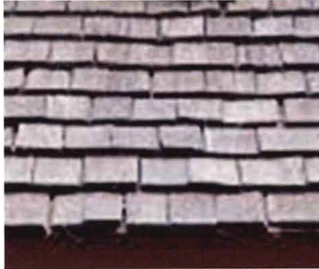
Wood shingle roof
