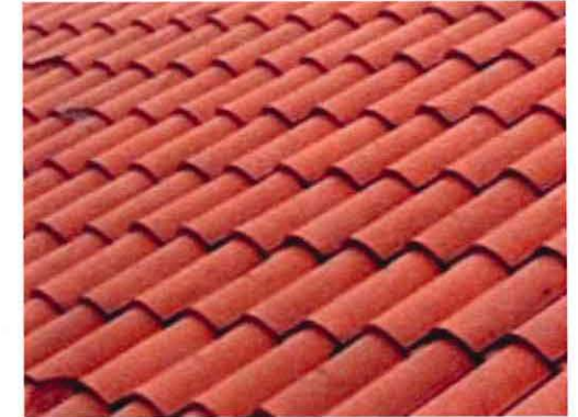
Clay tile roof
