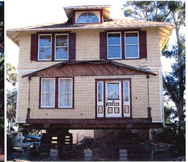
Foundation (and porch) was removed to allow for the building to be elevated to a new floor height for a flood mitigation project.
