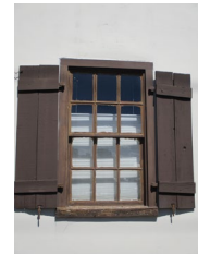
Window on the Front Elevation
