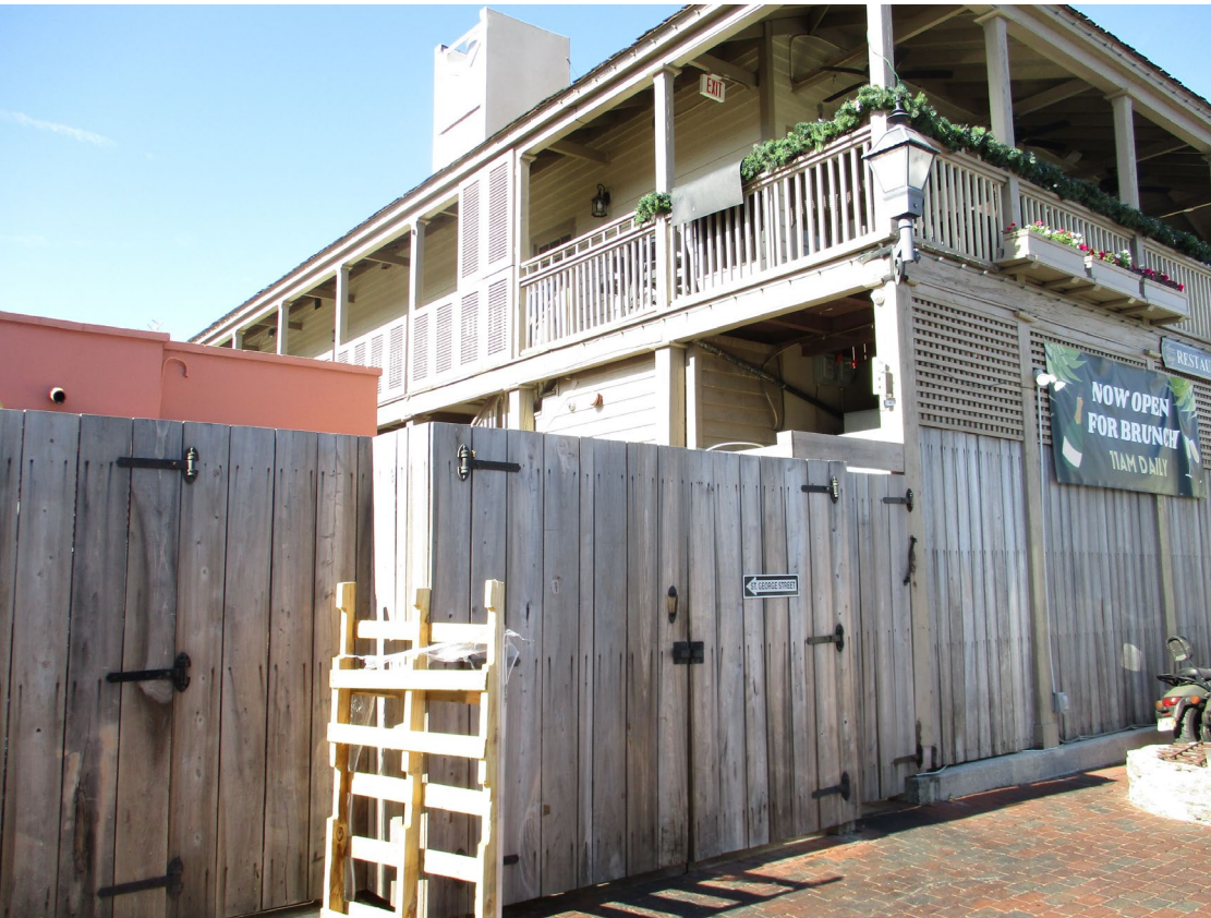
Rear of building: Facing northwest toward proposed location of project area behind wooden fence with adjacent building and fenced-in area to the north
