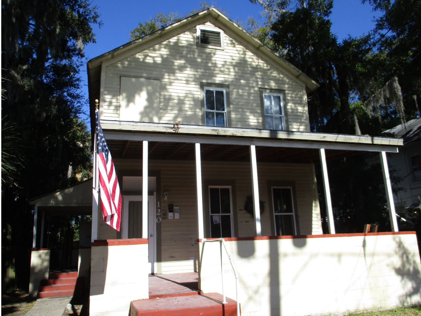
Front façade/south elevation of building, fronting Bridge Street: 2 nd floor door opening boarded up and is proposed to be returned to functional door
