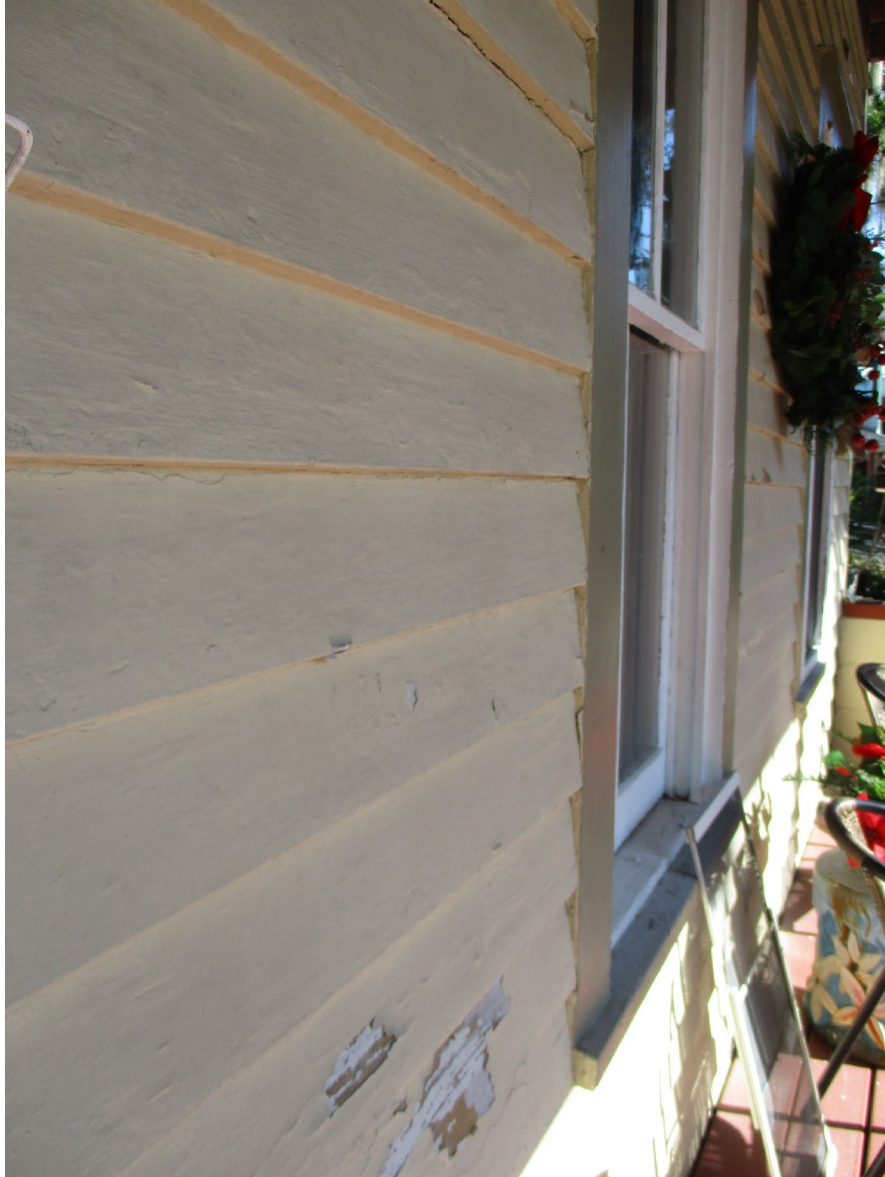
Historic wood lap siding proposed to be replaced with Hardie board type siding
