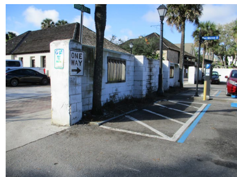
Parking Lot Side of Wall
