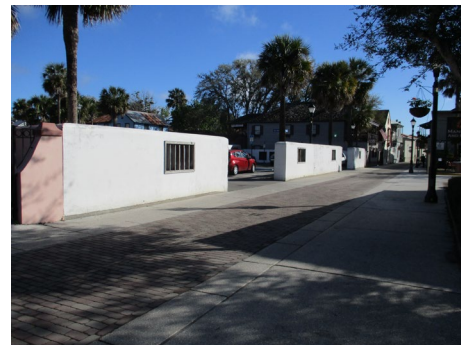
Street Facing Side of Wall
