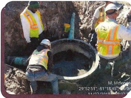
Workers install a manhole on Duero Street
