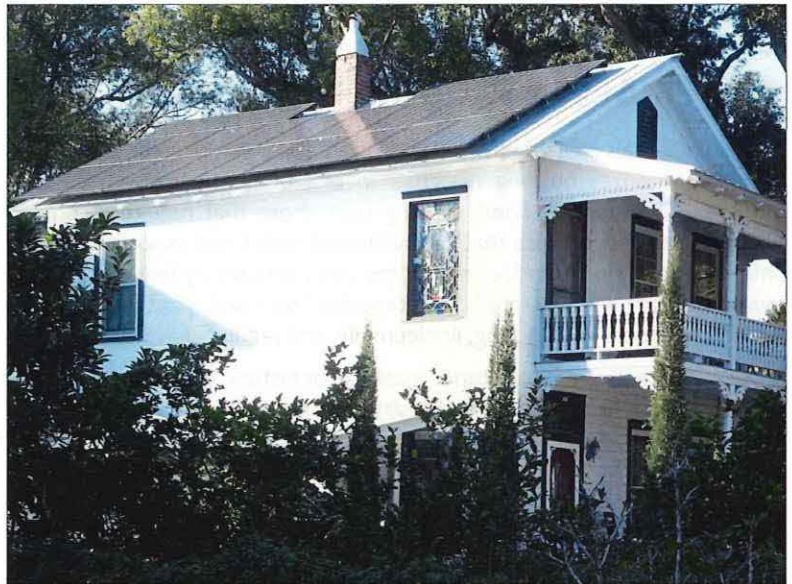
Secondary power sources, such as solar panels, can facilitate recovery from a flood. The visual impact of solar panels can be mitigated with placement on secondary elevations; installation parallel to the roof surface; selecting a frame-less panel that matches the roof color; and maintaining a consistent minimum offset of 6-inches from eaves, rakes, and ridges.
