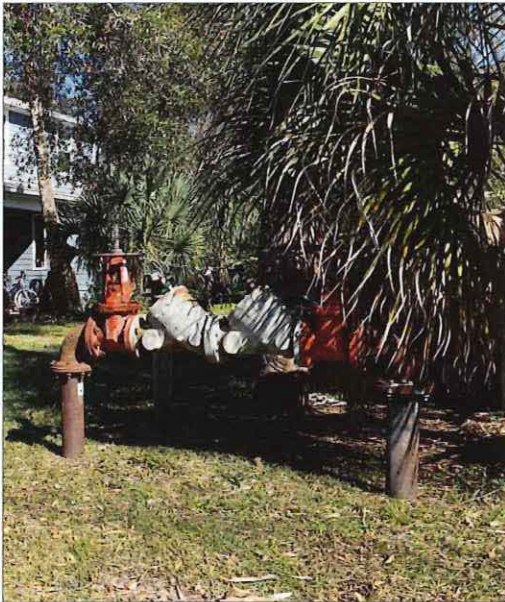
Municipal back flow preventers can protect contaminated water from entering the water supply in a neighborhood. Individual property owners can also install back flow preventers at water lines to protect their homes.
