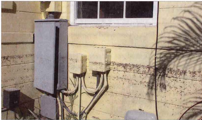
The height of the floodwater impacted the electrical service for this house. (Photograph courtesy of the City of St. Augustine.)
