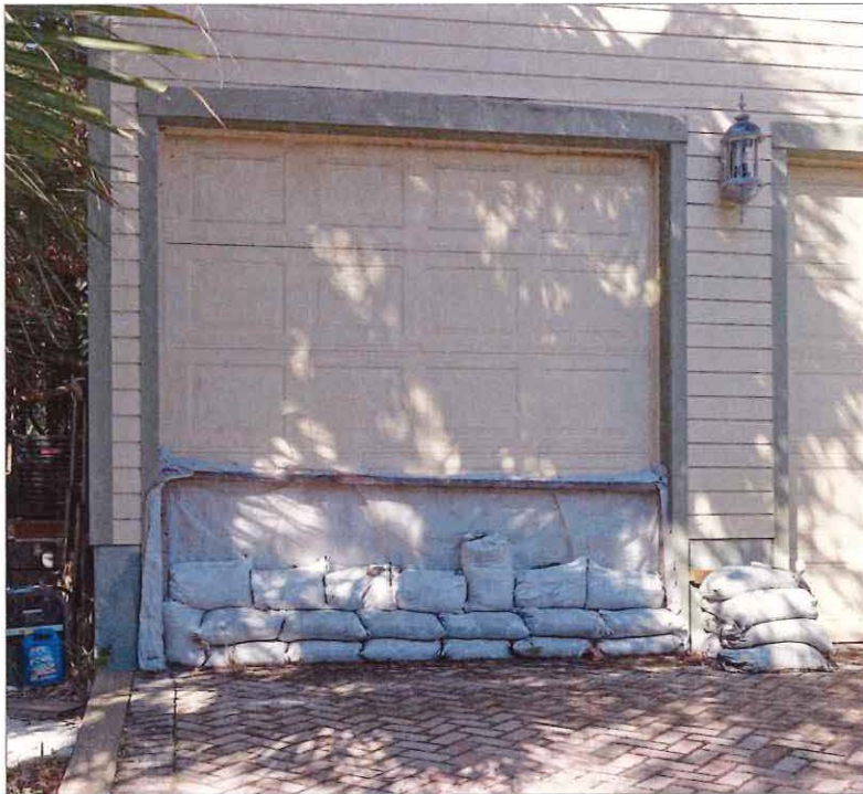
Sandbags are often used as part of a barrier system to reduce or prevent floodwater from entering through doors and windows. They must be properly installed to be effective, and treated as hazardous waste if they come in contact with floodwater.
