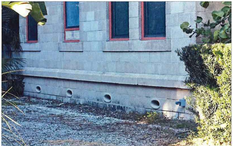
The size of the building and area of free water flow of the flood openings is key to determining the number of required flood vents. When proposing the installation of a non-traditional flood opening, care should be taken to verify there is adequate water flow.
