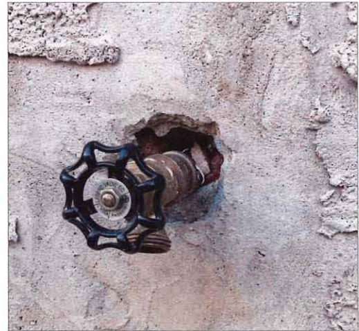
Sealing opening around penetrations such as hose bibs is recommended to reduce floodwater seepage, particularly if a barrier or shield system will be employed to minimize floodwater damage.
