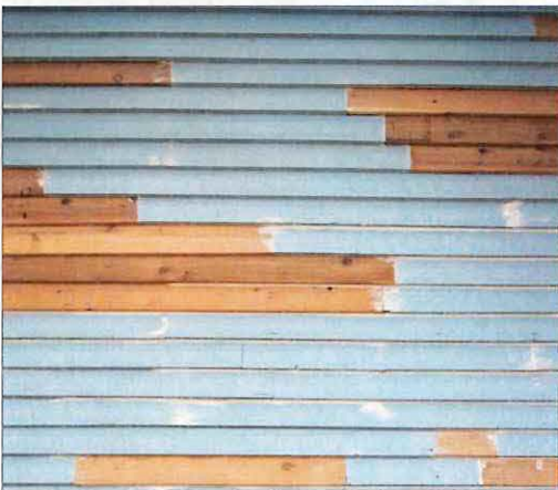
Replacing damaged or missing siding can prevent stormwater infiltration and prevent it from becoming airborne debris.
