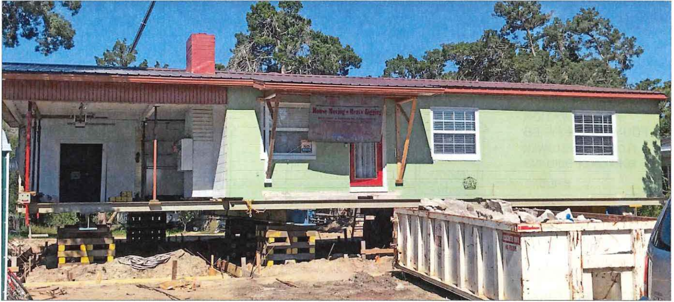
Slab-on-grade ranch houses, and their chimneys, can be successfully elevated. Care should be taken when addressing the raised foundation. (Photograph courtesy of the City of St. Augustine.)
