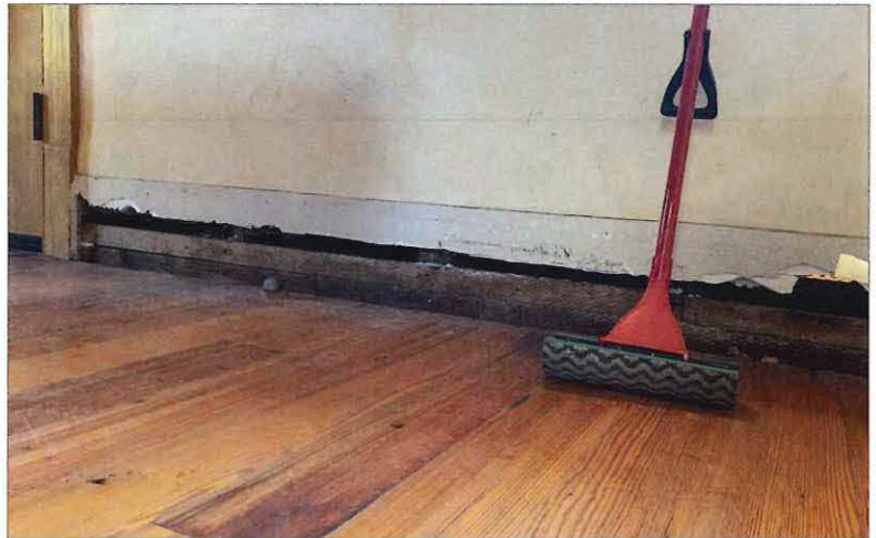
Removable baseboards and cornices can help dissipate standing interior water and promote air circulation, thus reducing the potential for mold.
