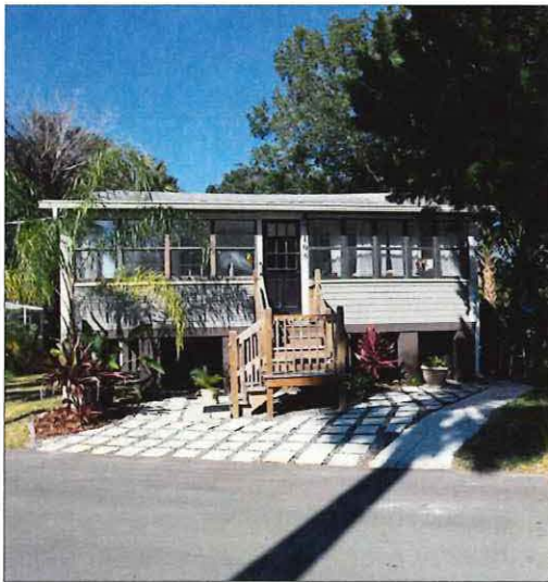
This one-story house has been elevated on piers. The piers and building base have been painted dark brown, reducing their visibility. The spaced driveway pavers allow for stormwater absorption.
