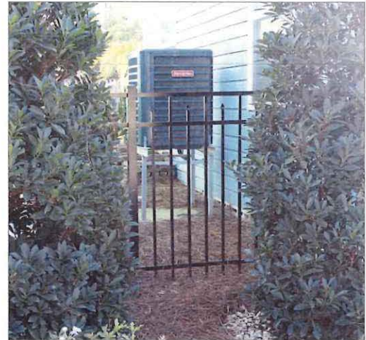
Exterior equipment should be installed so that it is elevated above the anticipated floodwater height. As the shrubs grow, they will provide visual screening.
