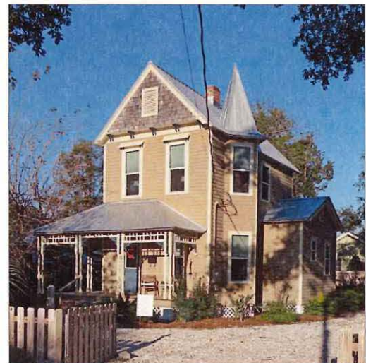
Queen Anne houses, which often include towers, chimneys and porches, can be more challenging to elevate than buildings with simpler geometries.
