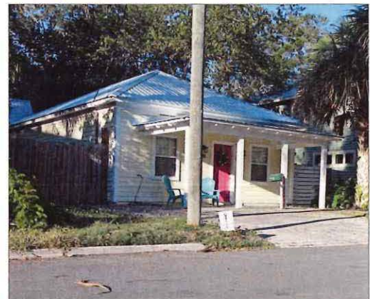
Buildings whose first floors are located close to the surrounding ground level are more vulnerable to flooding than neighboring buildings on piers.
