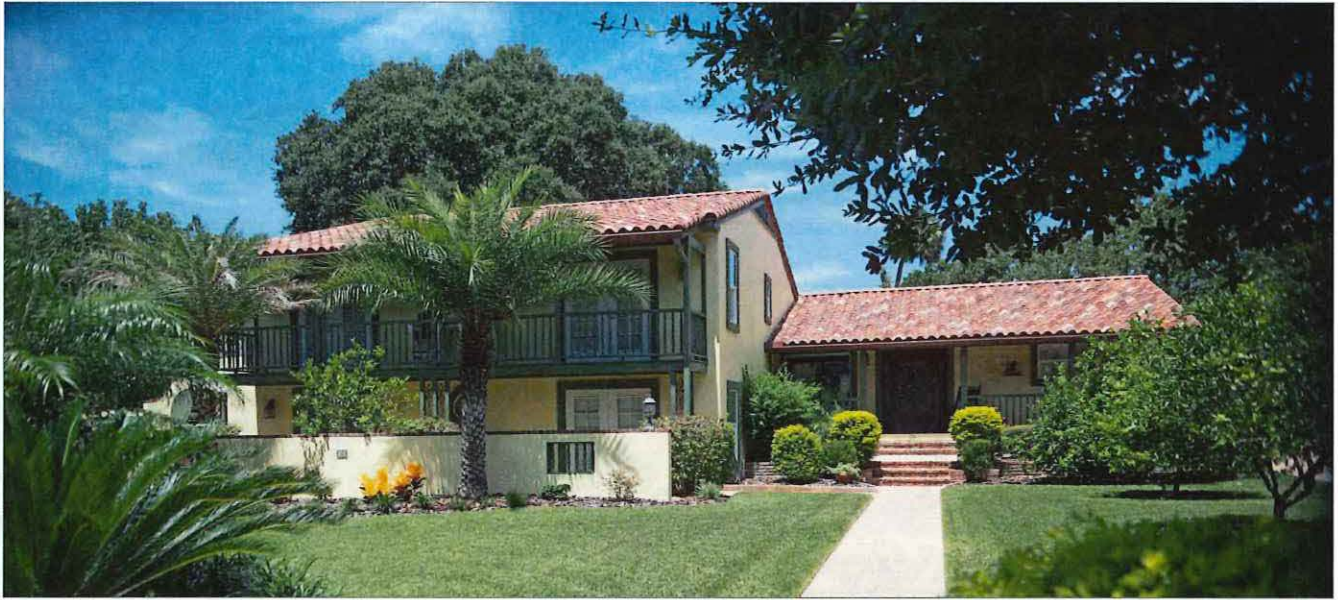
This home has three levels, two in the main block and an intermediate level at the one-story section to the right. The lower level of the main block is most vulnerable to flooding and it could be wet floodproofed. Wet Floodproofing would include relocating any systems or equipment to a higher level.
