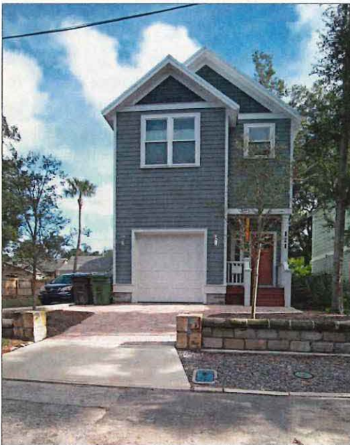
New residences constructed in flood-vulnerable locations are often wet floodproofed. To the extent possible, the form, scale, and materials of new construction should be compatible with neighboring existing buildings. This example includes a small front porch at the entry. In addition, the site has been raised, reducing its flood vulnerability. Flood impacts to adjacent properties should be mitigated.
