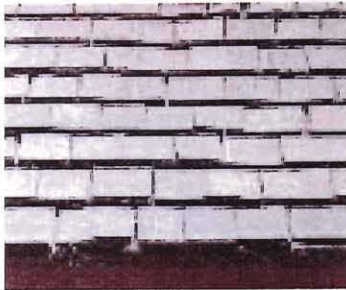
Wood shingle roof
