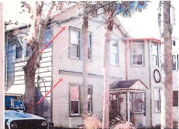
Evidence on the Sanborn map (left) and the building shows there used to be a historic two-story frame porch likely removed ca. 1930-1950s when asbestos siding was added. Reconstructing a compatible porch could be approved by staff.
