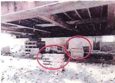
A building elevation project revealed unique coquina stone piers (background) along with traditional brick piers (foreground)
