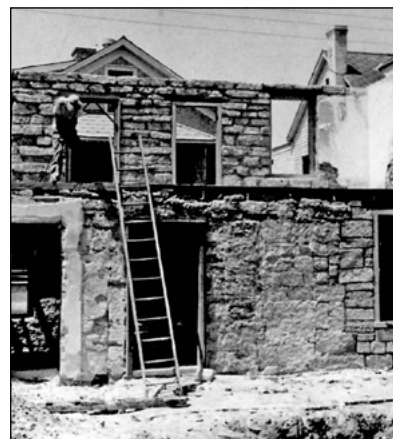
The rear of the Llambias House during the 1954 restoration. (National Park Service)
