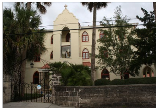
Sisters of St. Joseph Convent, 1874. The Mission Revival parapet is a later addition.
