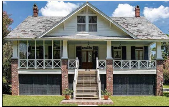
This house was elevated six feet, necessitating new stairs and piers. The historic porch materials were retained. The dark lattice below helps to visually tie the building to the ground. (National Park Service)
