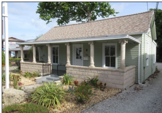
6 Perpall Street, 1916. Note the use of molded concrete blocks and columns for the porch.
