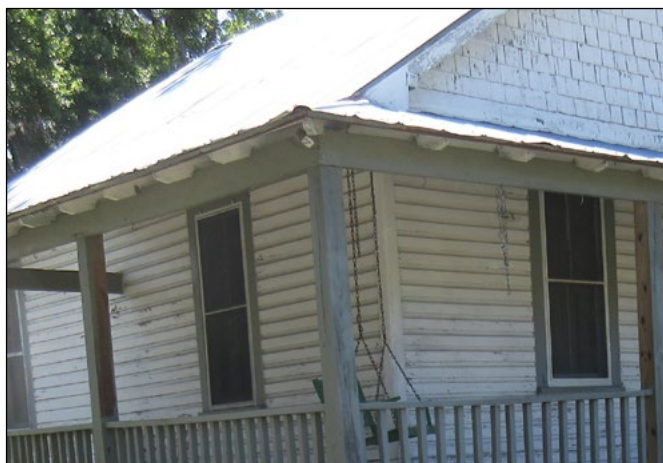
Wood shingles used in the gable end with novelty siding below.
