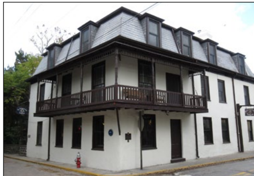
279 St. George Street, Garcia-Dummet House, built in 1791-1795 with a third floor addition in the Second Empire style.
