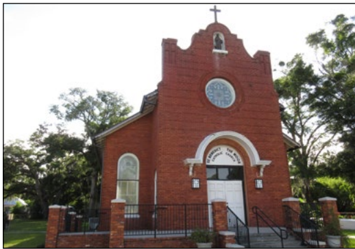
86 Martin Luther King Avenue, St. Benedict Catholic Church, 1915.
