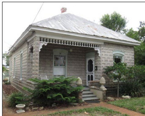
17 Cincinnati Street, built c. 1905 using cast concrete block.
