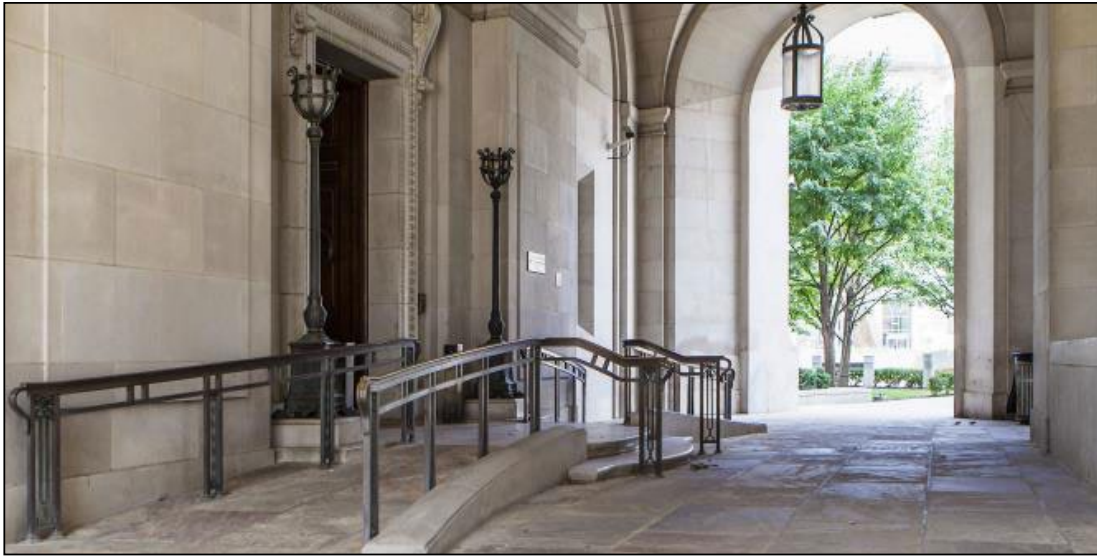
This accessible ramp uses materials that harmonize with the rest of the building.
