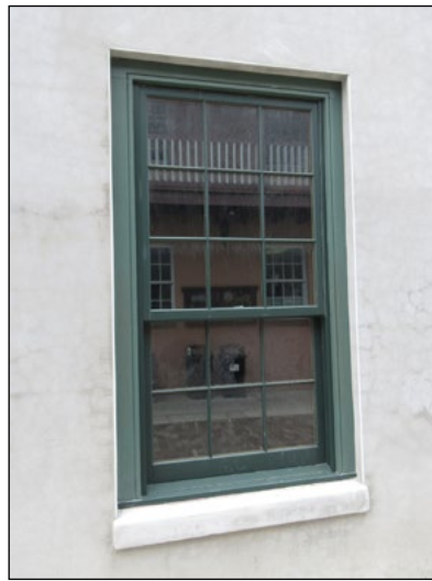
Historic wood window compared to an aluminum-clad wood window. Although similar, the profiles, depth, and textures of the historic window are more prominent.
