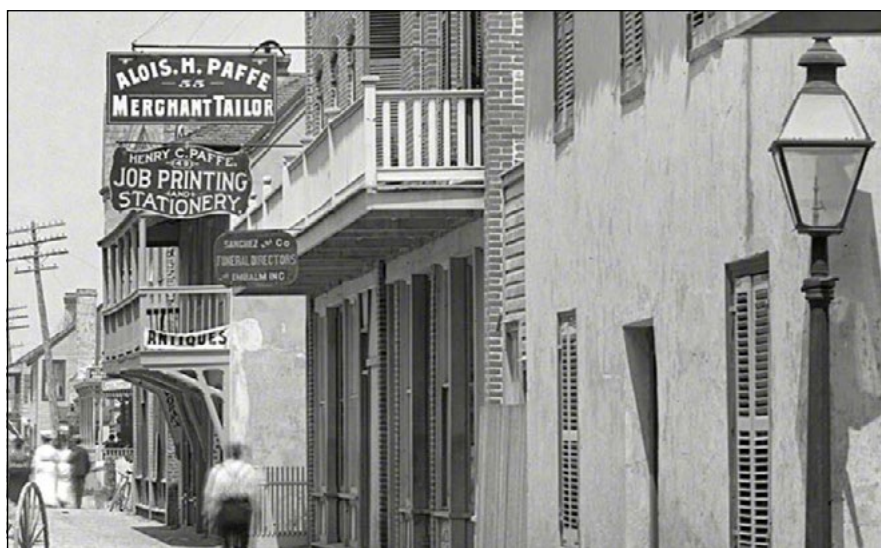
Signage along St. George Street, 1910.
