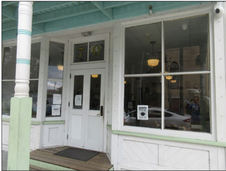
This storefront is typical of commercial design trends during the late 1800s and early 1900s.
