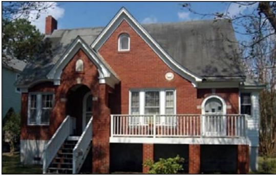
The front porch and entry were raised on concrete block piers which were veneered with brick. The main portion of the house rests on a new perimeter concrete block foundation. (FEMA)
