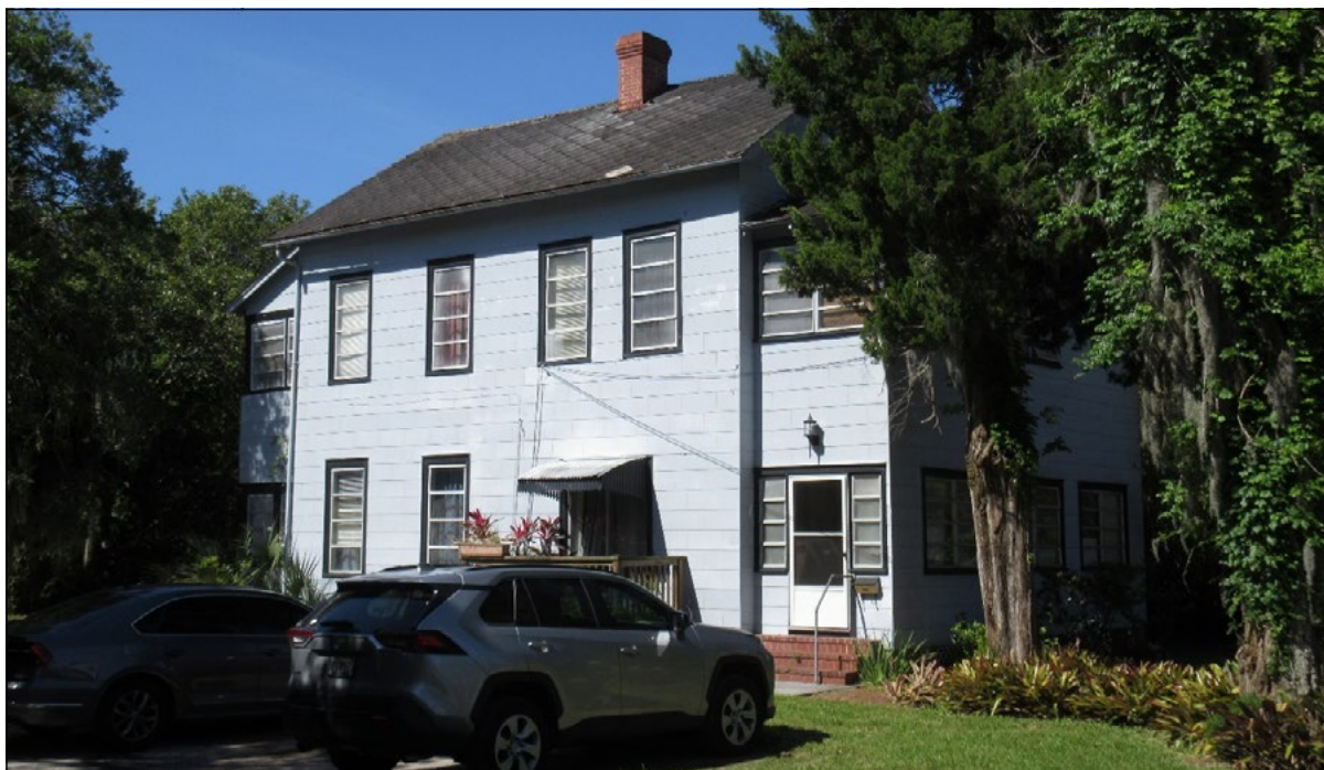
This building was previously altered by covering the wood cladding with asbestos shingles and replacing the original wood windows with aluminum windows. It could be a candidate for restoration.
