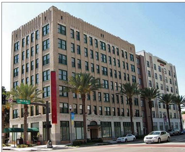
The addition at right draws from the historic window pattern and maintains the street rhythm.
