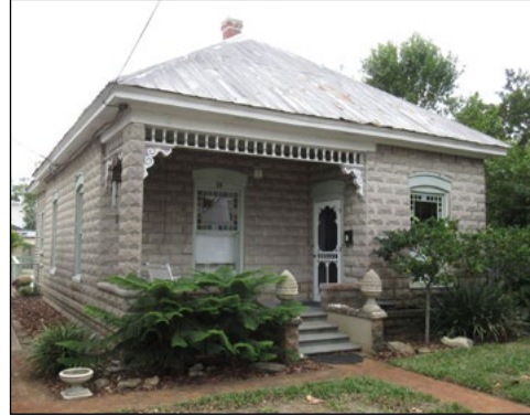
17 Cincinnati Street, built c. 1905 using cast concrete block.
