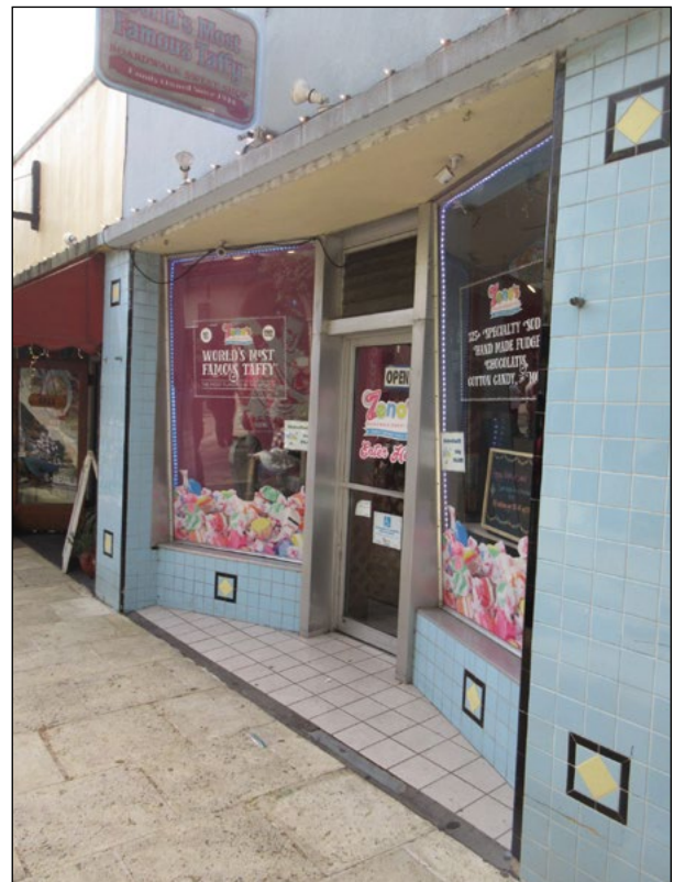
Aluminum storefront systems with angled walls and windows became popular during the mid-20th century.
