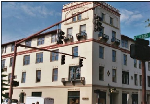
206 St. George Street, Lyon Building, 1886-1887.
