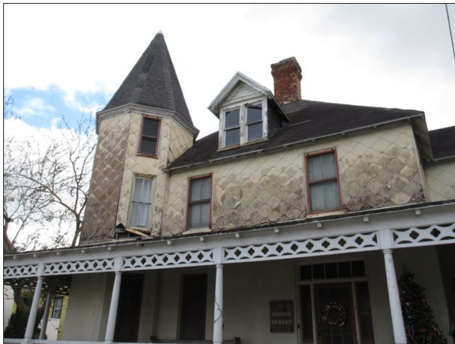
Asbestos shingles applied in a fish scale pattern to 11 Bridge Street.
