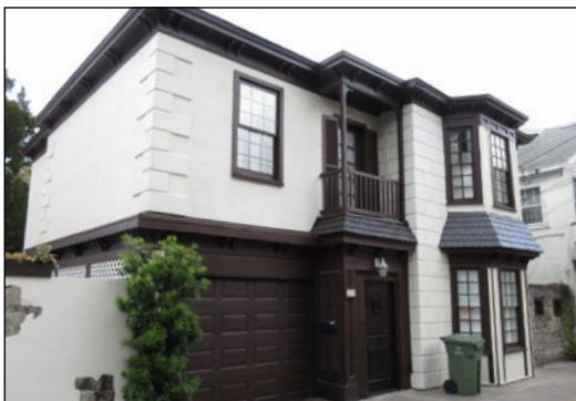
34 St. Francis Street, 1885-1893. Note the quoins on the building corners.
