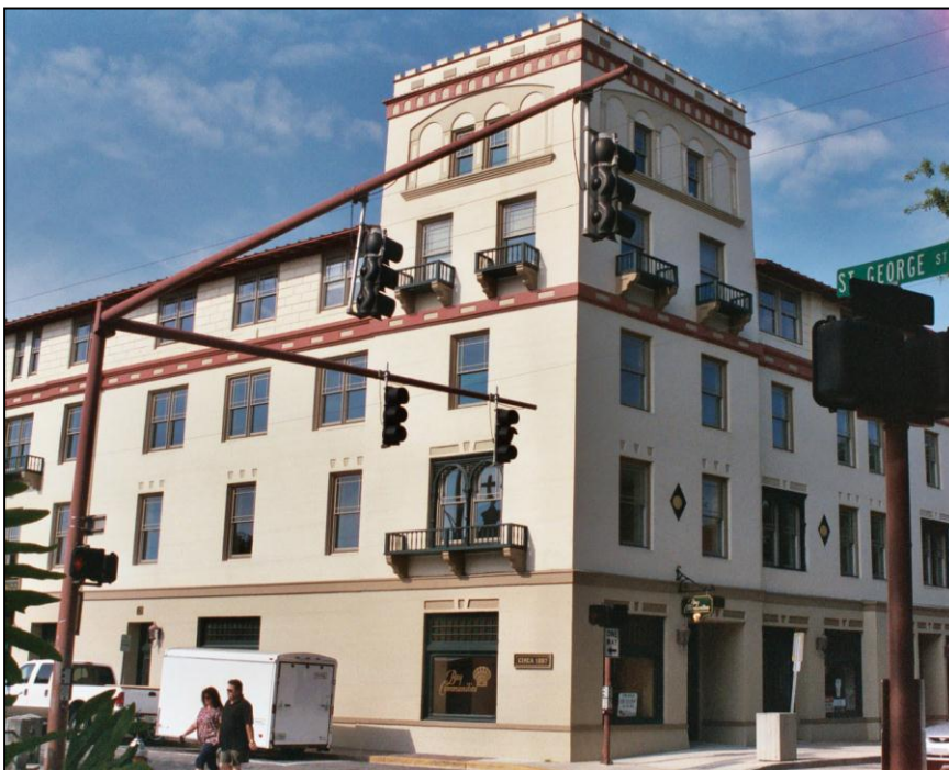
206 St. George Street, Lyon Building, 1886-1887
