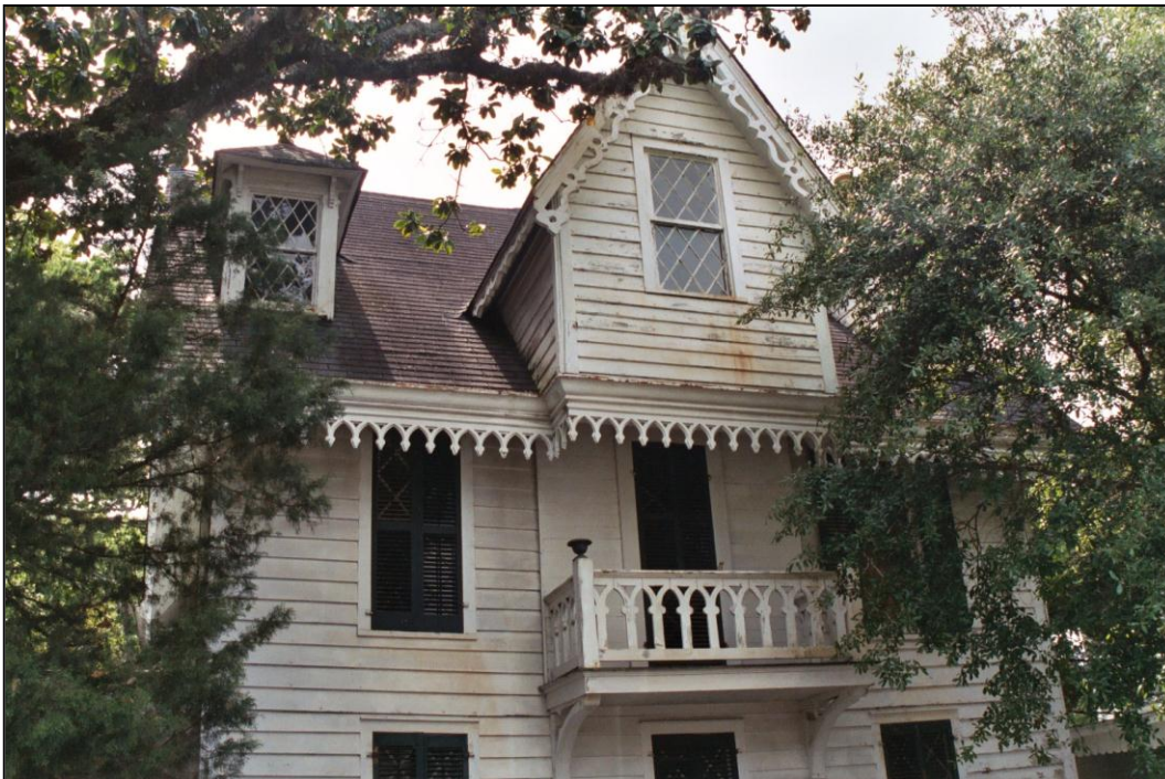
232 St. George Street, Stanbury Cottage/ Gingerbread House, 1857-1869
