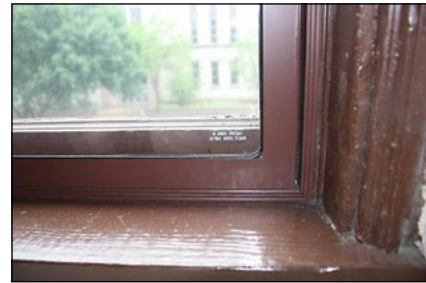
Interior storm windows can improve energy efficiency without changing the exterior look of your historic windows. (National Park Service)
