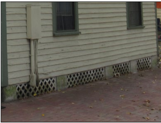
Lattice should be placed between piers. However, the lattice should also be placed at a 90 degree angle.
