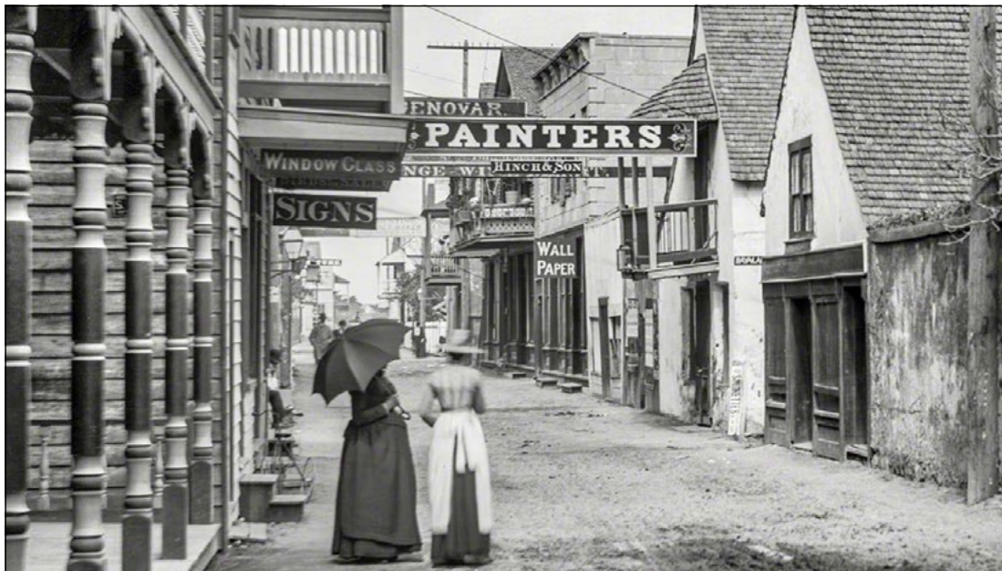
Signage along St. George Street, 1894.
