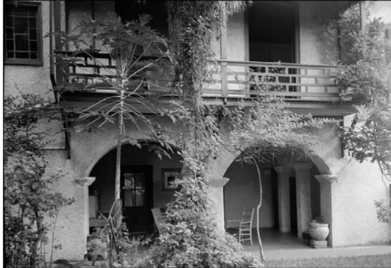
Loggia and balcony of the Don Pedro Horruytiner House, 214 St. George Street.
