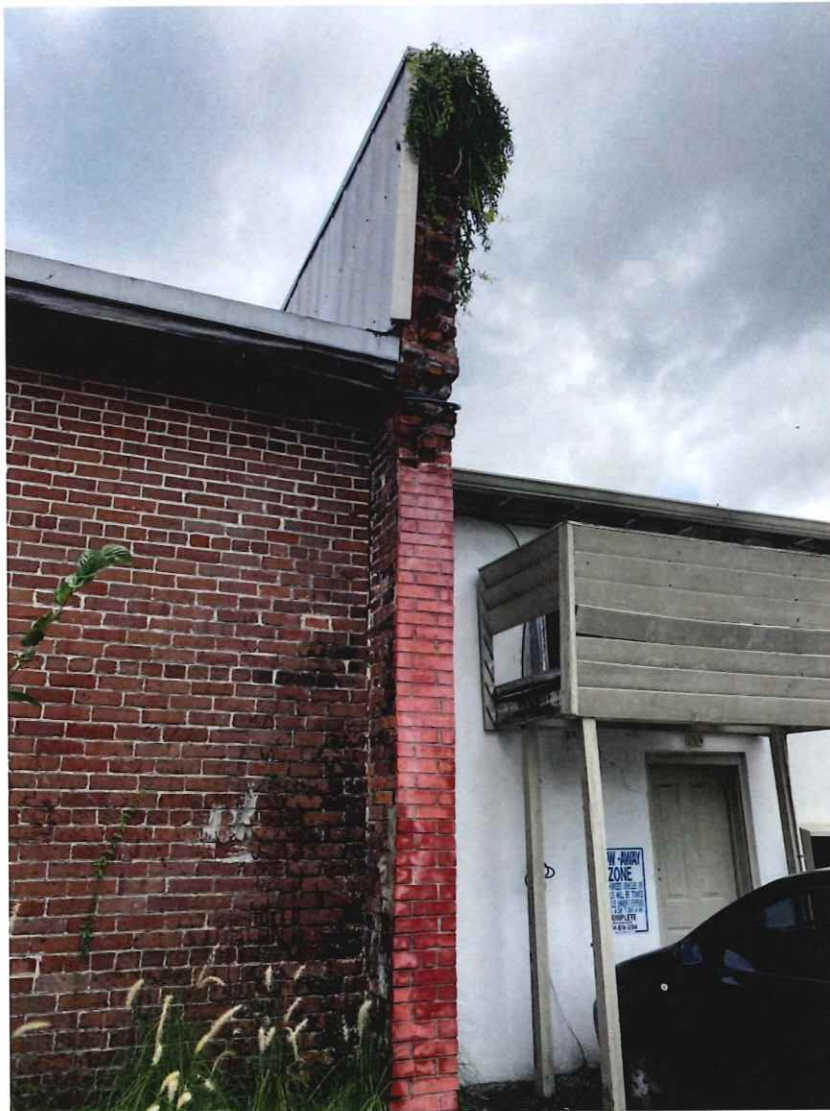
Photo 1.06 - Wall from Alley
