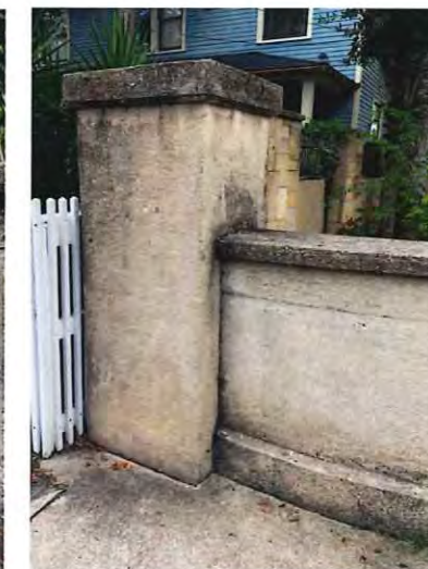
Rammed concrete wall at Sisters of St. Joseph constructed circa 2005
