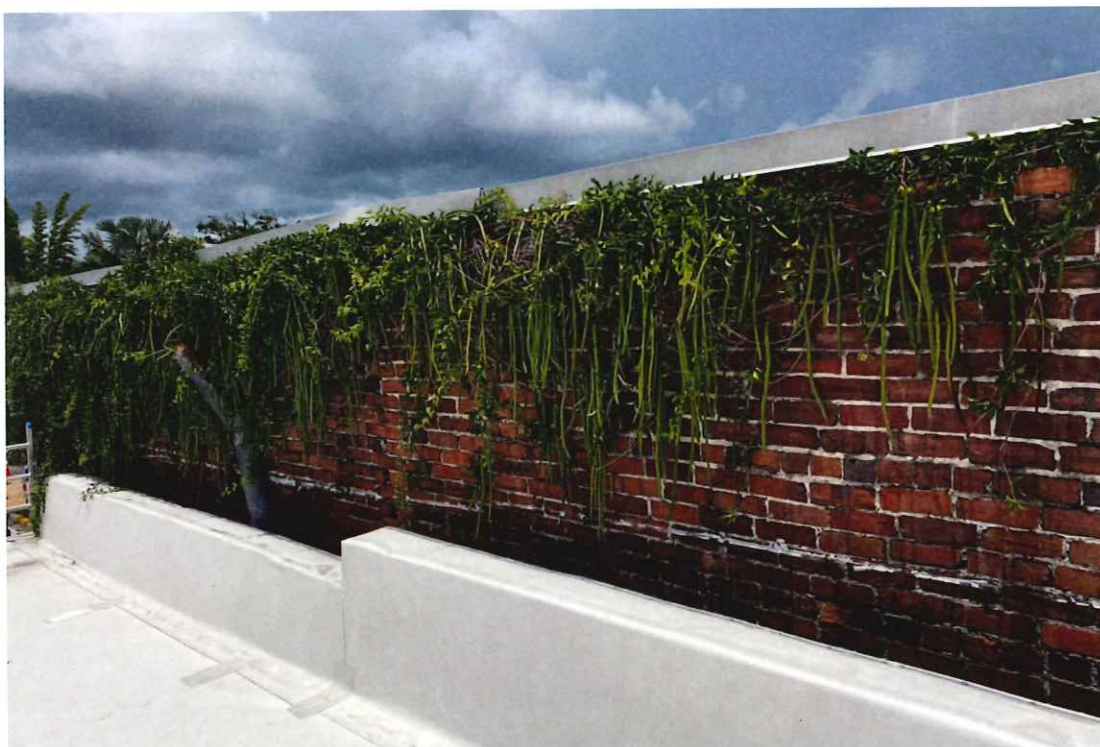
Photo 1.04 - Wall from roof of adjacent building
