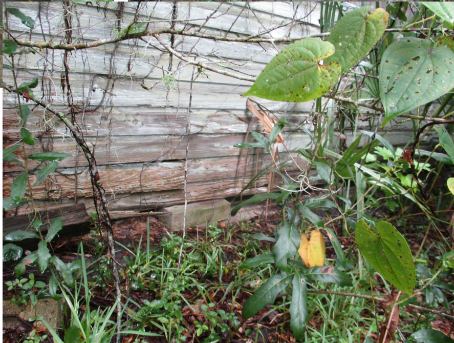
South Elevation: Looking north
