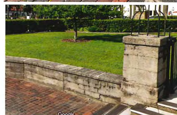
Existing rammed concrete columns and site walls on the Lightner grounds which will be matched for perimeter wall
