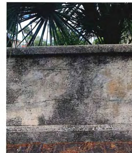
Rammed concrete wall at Sisters of St. Joseph constructed circa 2005
