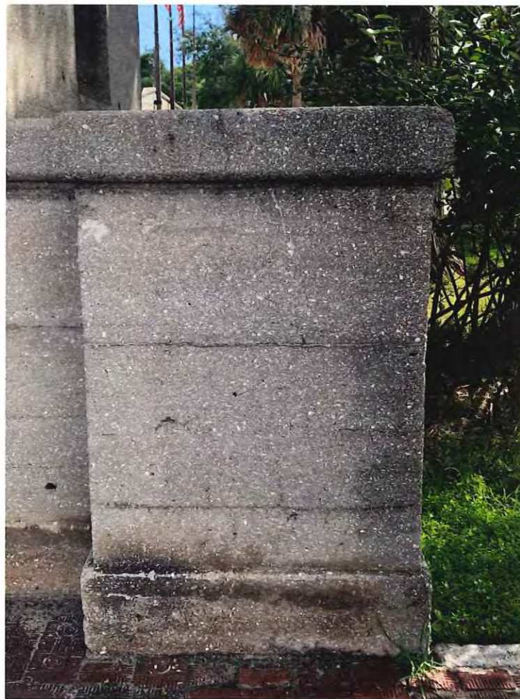
Existing rammed concrete columns and site walls on the Lightner grounds which will be matched for perimeter wall
