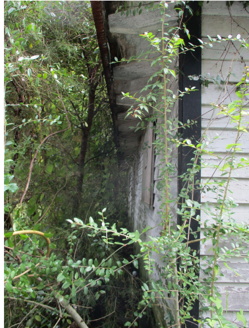
North Elevation: Looking east
