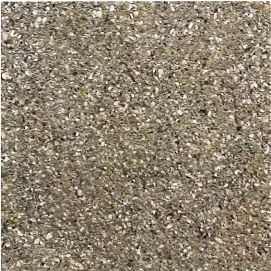
Coquina concrete (seawall)
