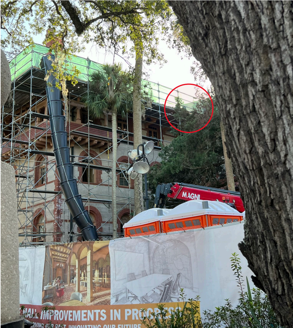
South Elevation East Wing (behind scaffolding) Paired Window Sashes to be replaced with aluminum
