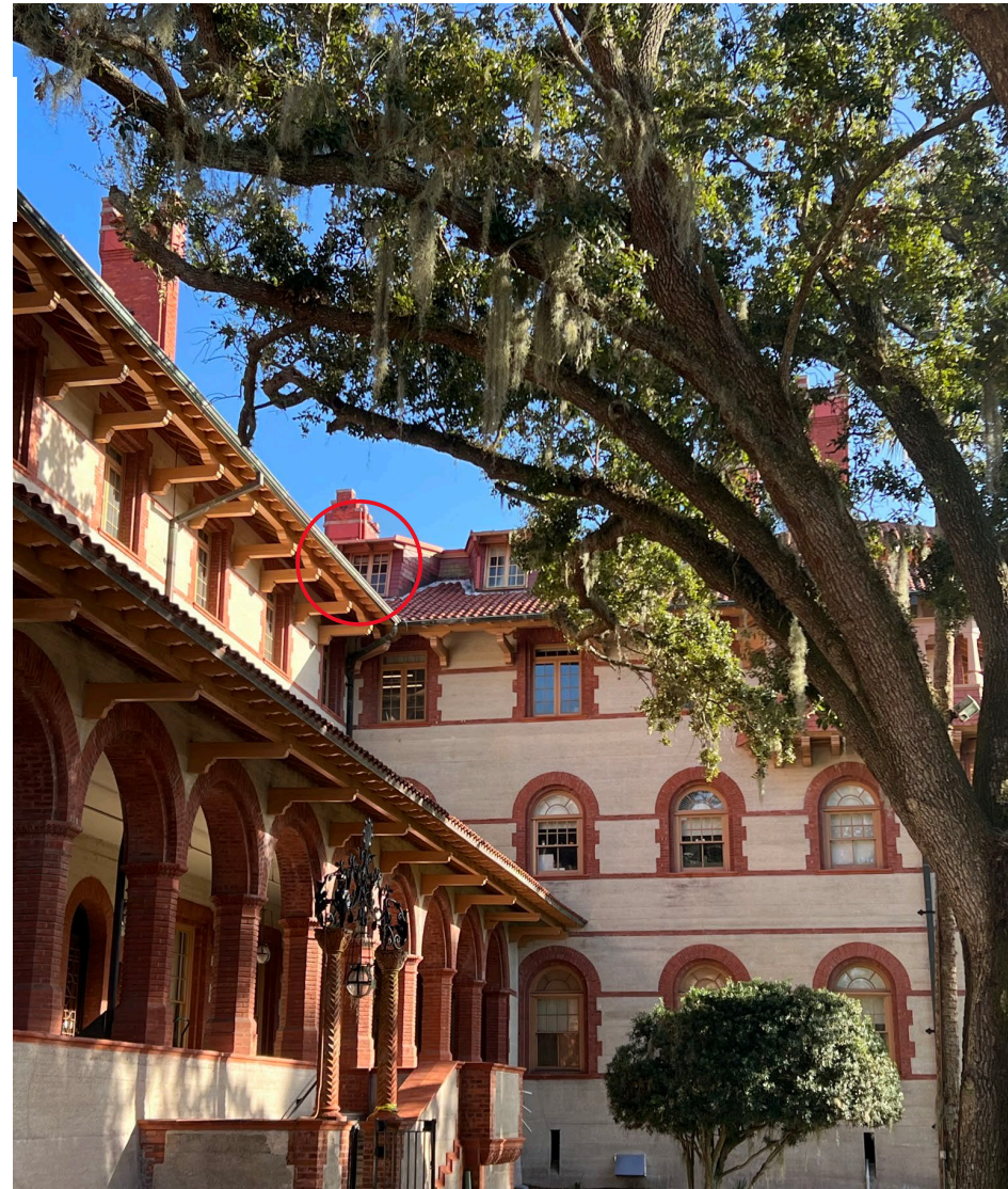
South Elevation West Wing Paired Window Sashes to be replaced with aluminum
