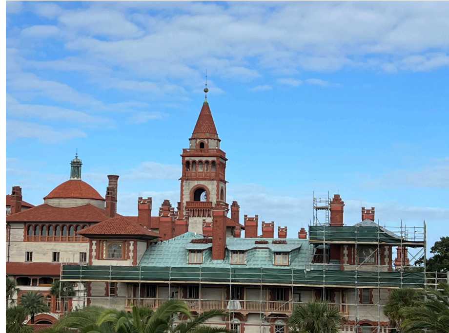
Vent and Exhaust in Tower
