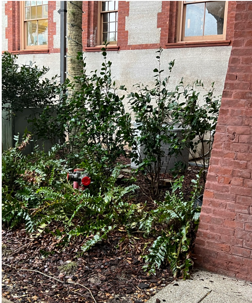
South Elevation East Wing Existing HVAC unit screened with plants (location of new piping and conduit)
