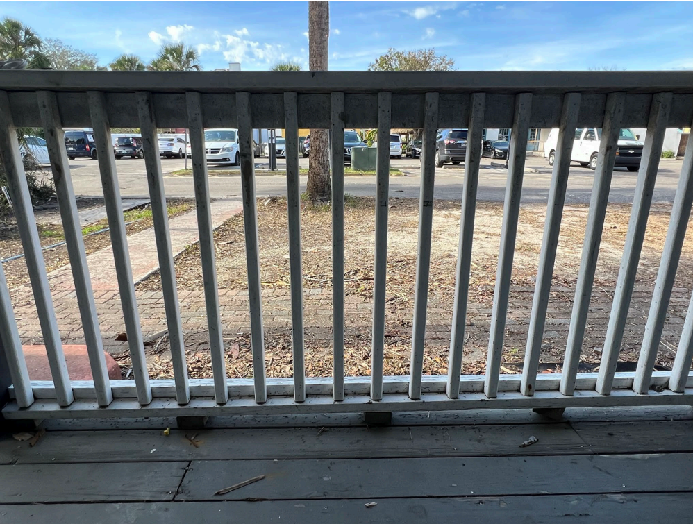
Existing wood porch railing and siding on front façade/west elevation – December 2022
