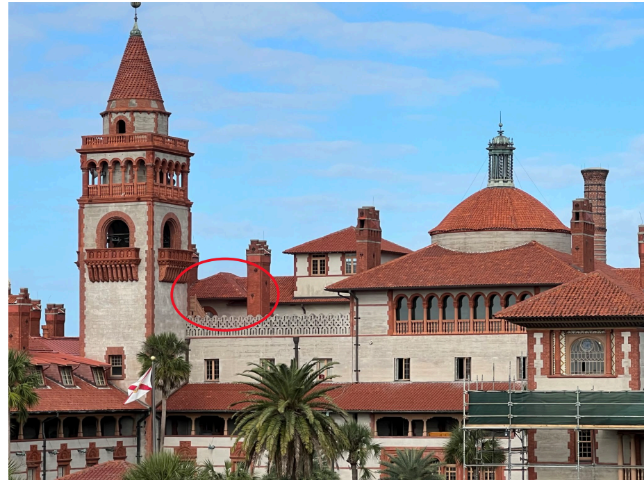
Vent under overhang of roof
