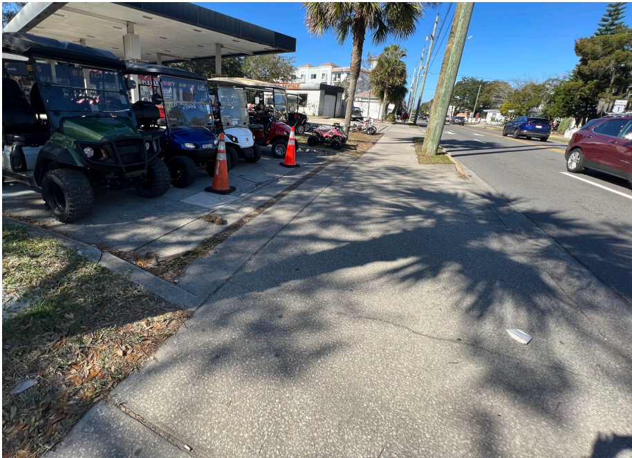
Existing Driveway Apron from San Marco Proposed for Removal (foreground)
