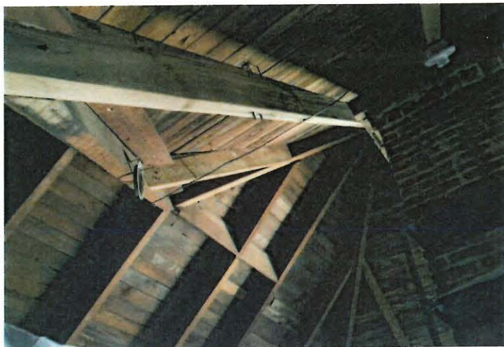
Image 11: High Roof Framing from Attic Access
