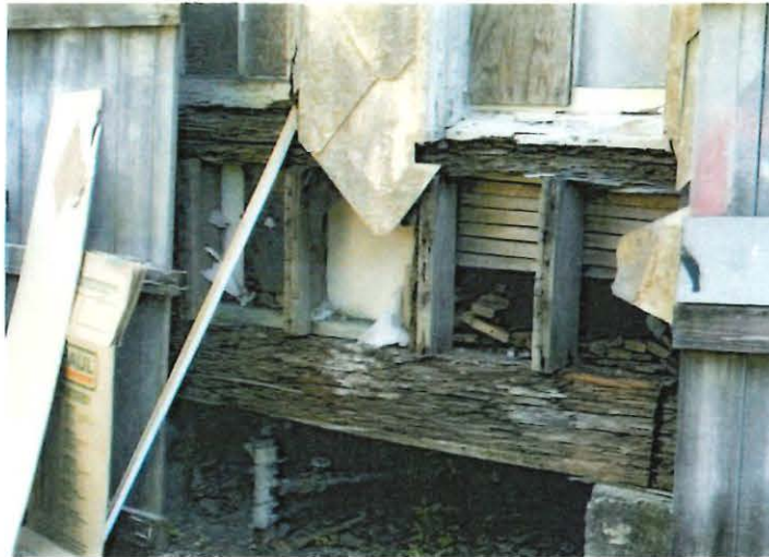
Image 5: Exposed Floor Beam and Wood Studs
