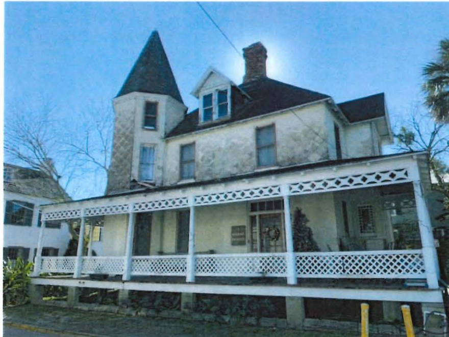
Figure 1: Front View of Structure
