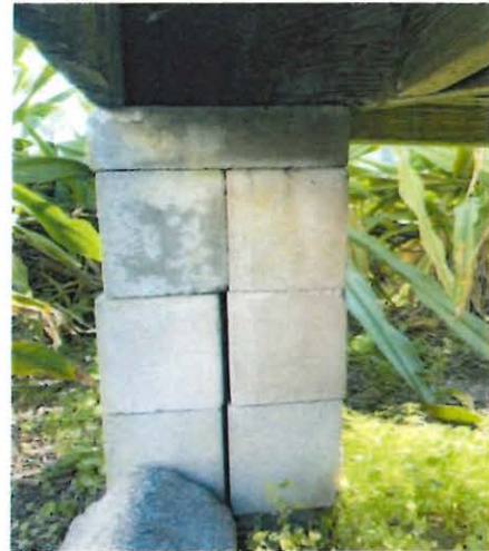
Image 2: Hollow Block Stacked Pier
