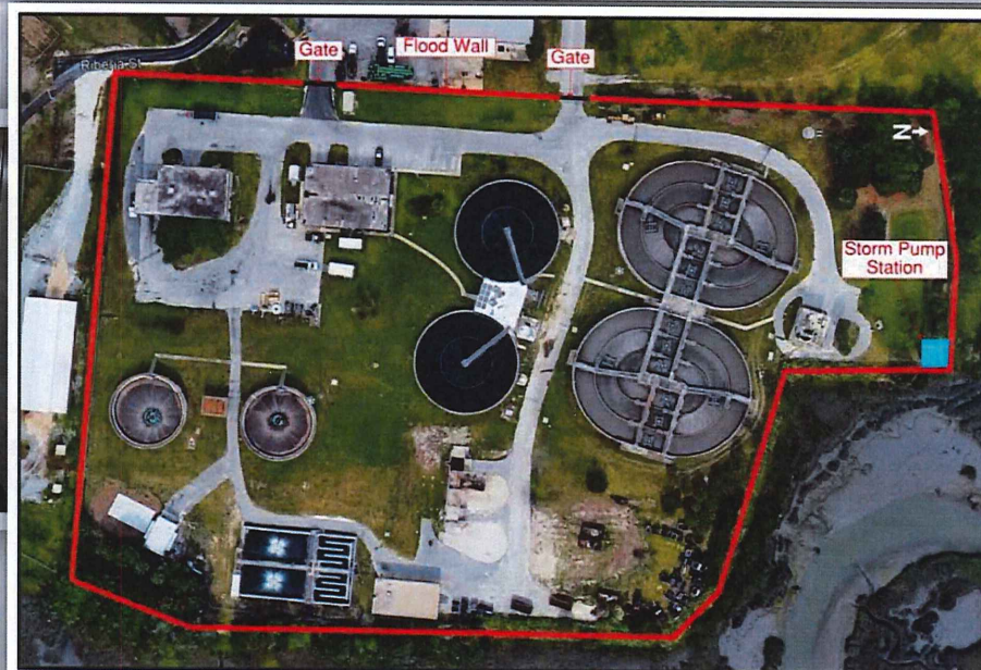
Figure 10: Perimeter Flood Wall and Pump Station
