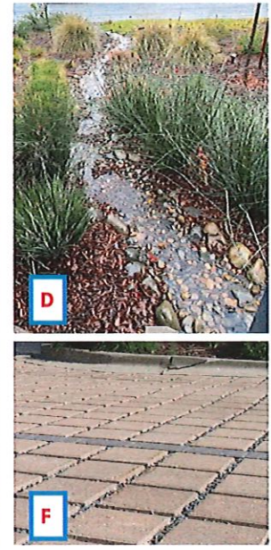
Examples of Stormwater Facility Design
