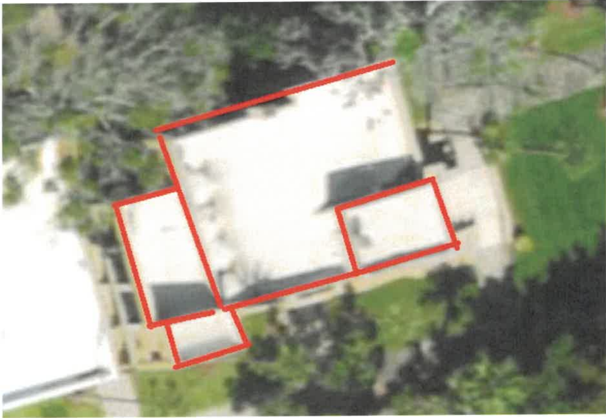
Figure 1. Areas to be repaired.
