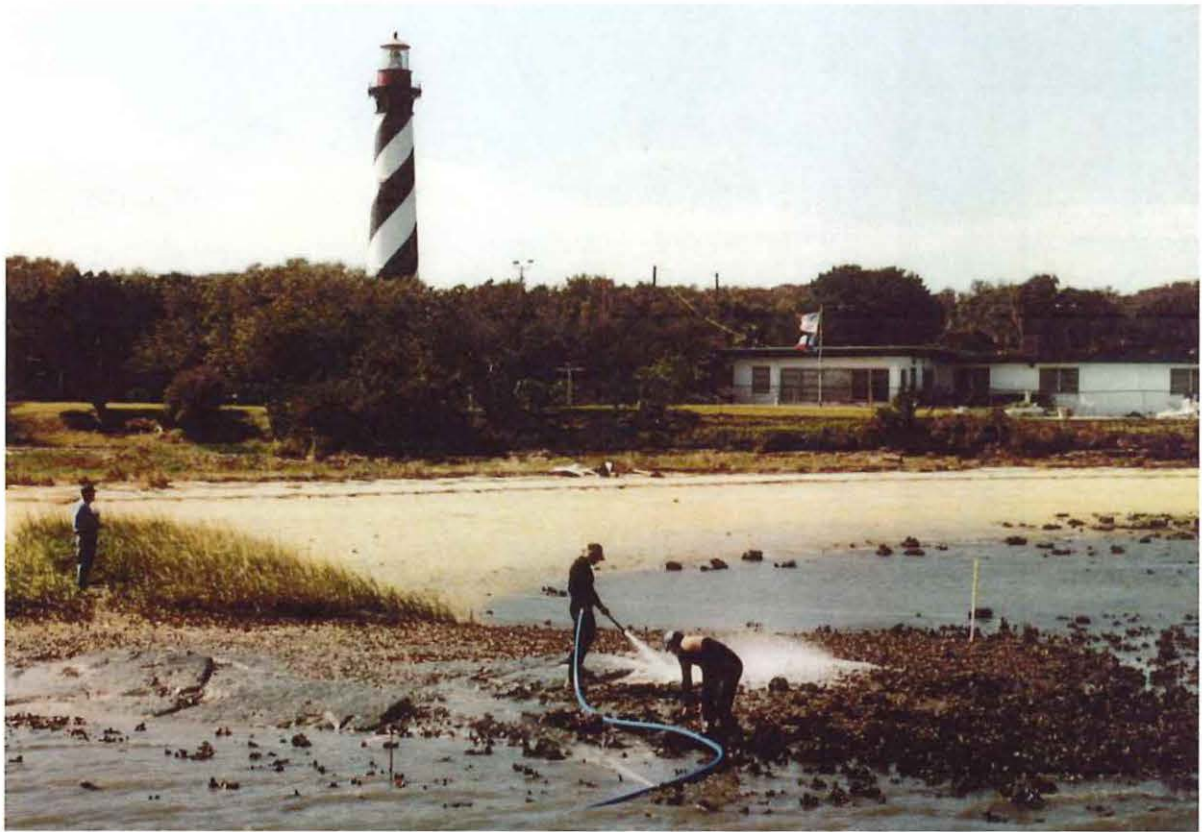
Figure 23. Cleaning the Old Lighthouse/Watchtower foundation stones of mud during LAMP's 2002 investigation of the site. Photograph courtesy of LAMP.
