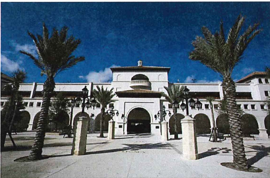
HISTORIC DOWN TOWN PARKING FACILITY Multi-modal Transportation Facility
