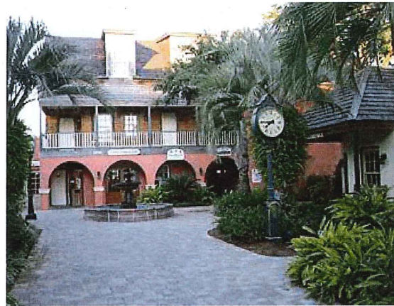
CITY GATES PLAZA THREE SECOND SPANISH PERIOD BUILDINGS DESIGNED AROUND A COURTYARD
