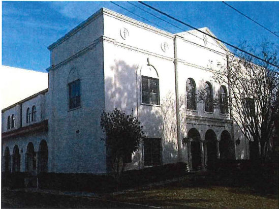
BISHOP BAKER PARISH CENTER CATHOLIC CHURCH MULTI-PURPOSE HALL
