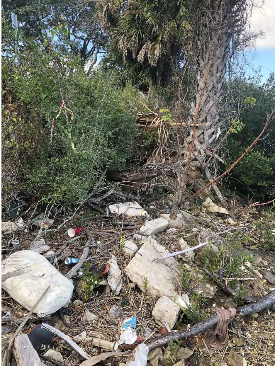
Figure 6 - Existing rip-rap shoreline (cont.)
