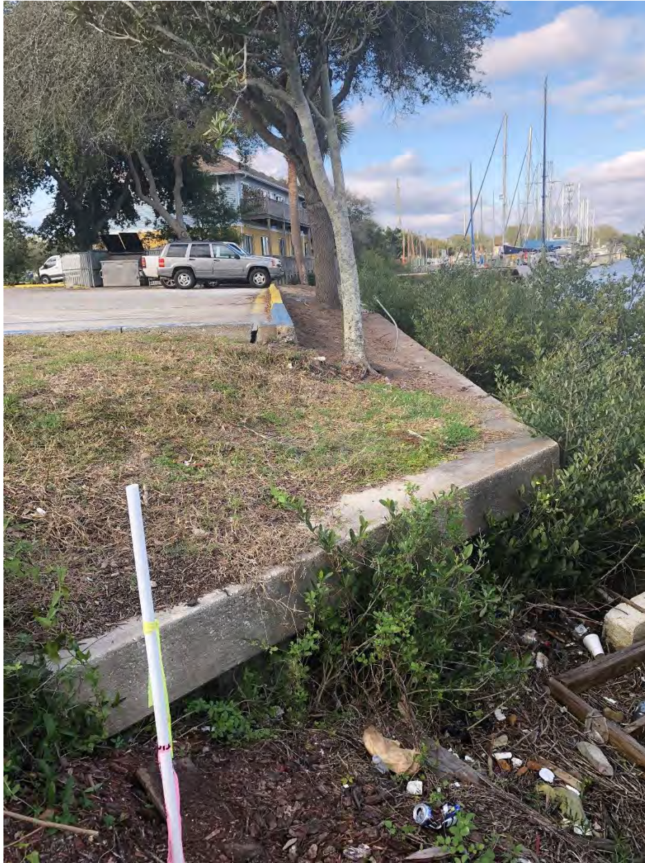
Figure 1 - Northern concrete bulkheaded boundary
