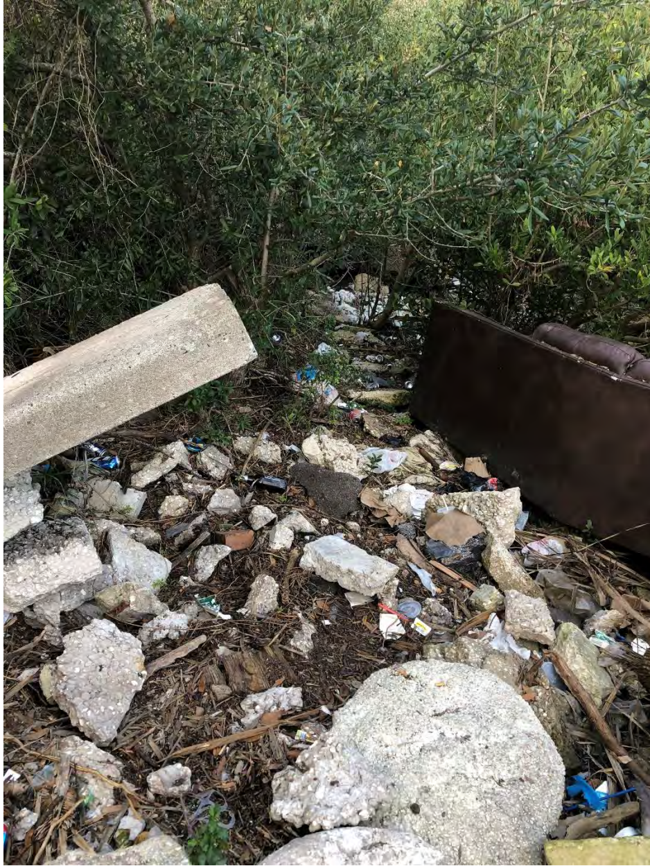
Figure 9 - Existing rip-rap shoreline (cont.)
