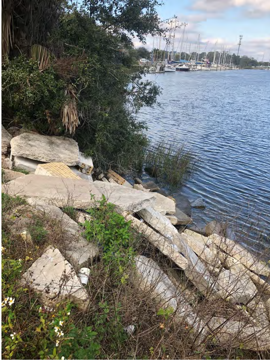
Figure 4 - Existing rip-rap shoreline (cont.)
