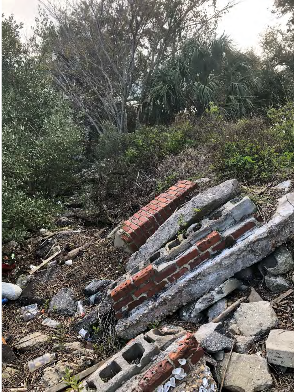
Figure 5 - Existing rip-rap shoreline (cont.)
