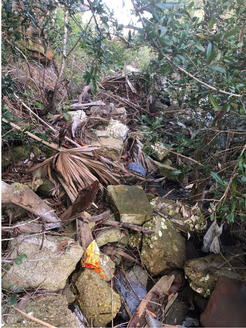
Figure 8 - Existing rip-rap shoreline (cont.)
