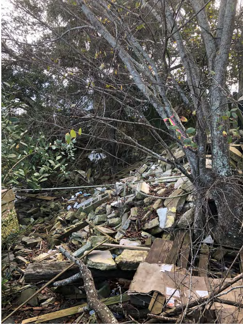
Figure 7 - Existing rip-rap shoreline (cont.)
