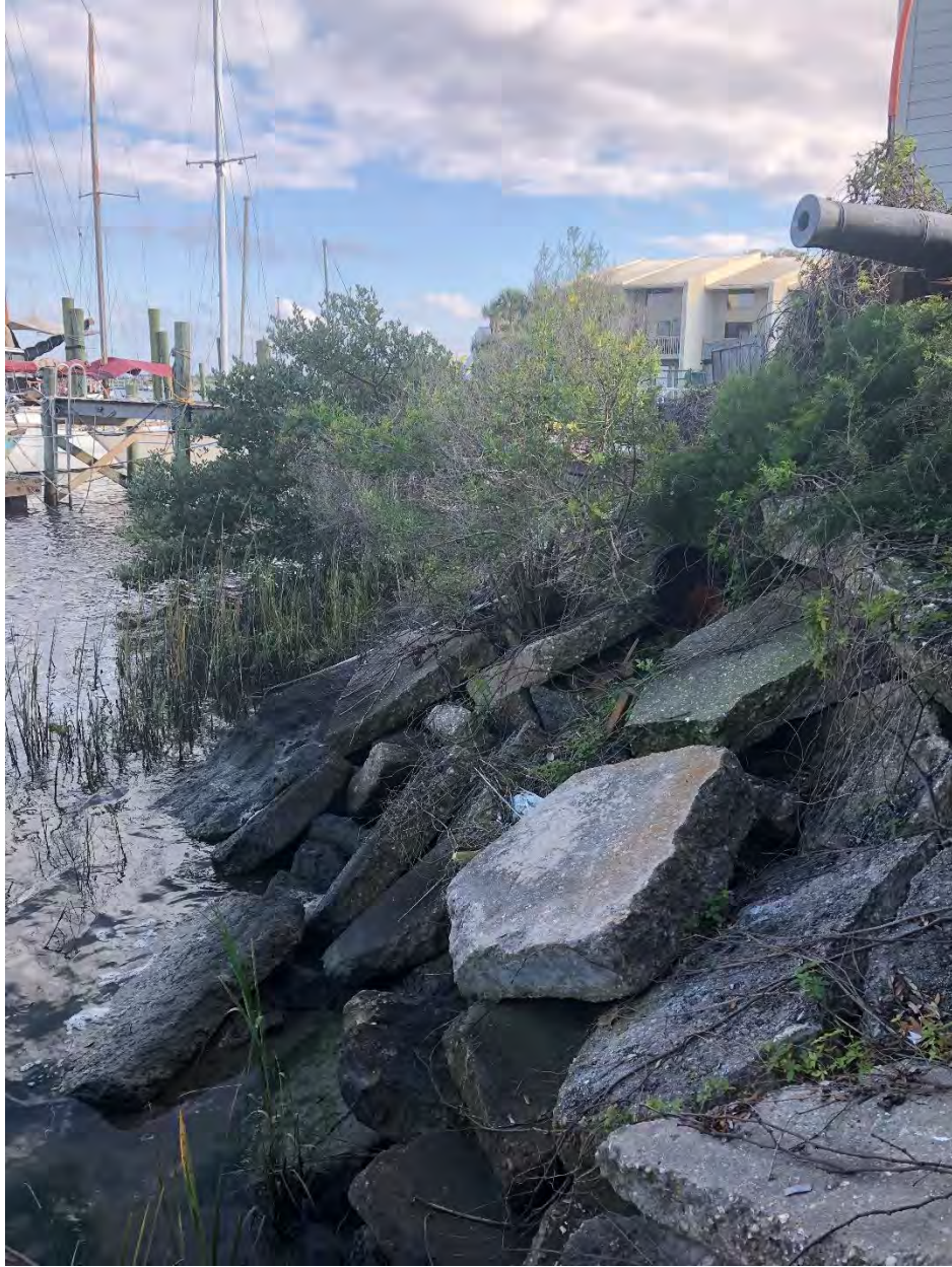
Figure 3 - Existing rip-rap shoreline
