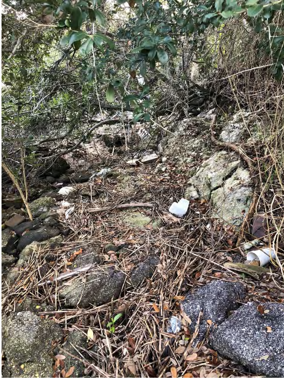
Figure 10 - Existing rip-rap shoreline (cont.)
