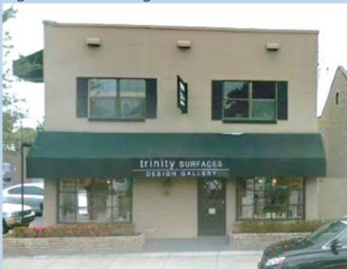
Prohibited (across several windows)
