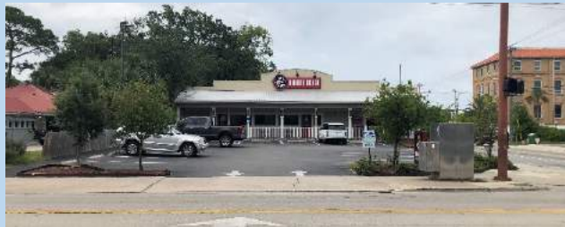
Figure 23: Examples of Existing Non-Conforming Parking Facilities
