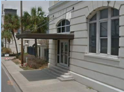
Figure 17. Example of Canopies
