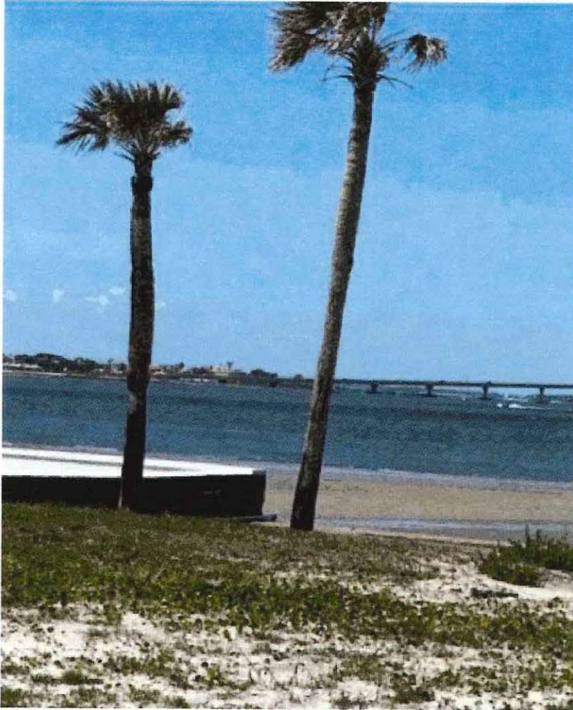
SOUTHERN END BULKHEAD NEIGHBORING BULKHEAD APPROXIMATELY 2.5' ELEVATION
