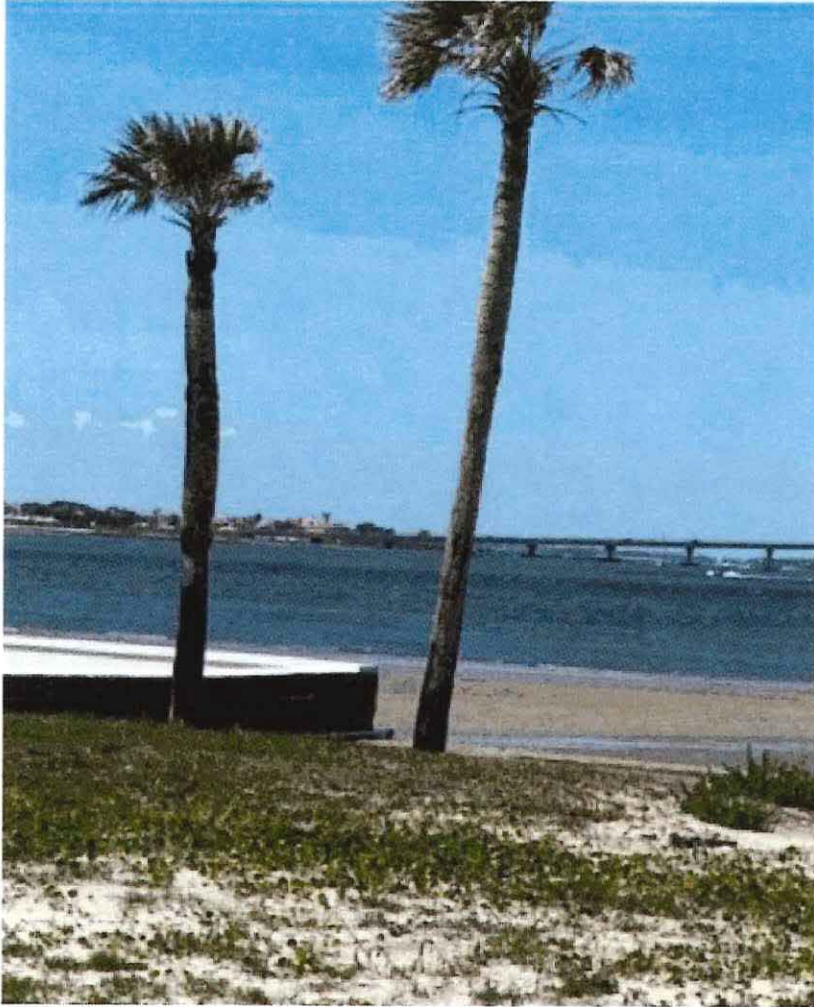
SOUTHERN END BULKHEAD NEIGHBORING BULKHEAD APPROXIMATELY 2.5' ELEVATION
