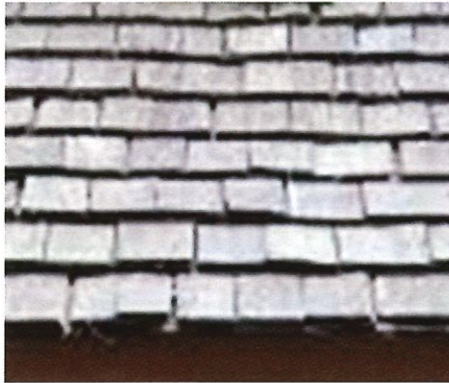
Wood shingle roof
