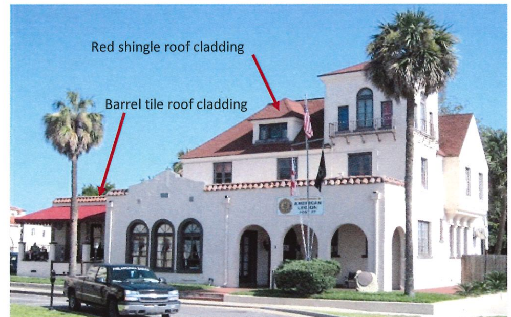
Stamped metal shingle roof
