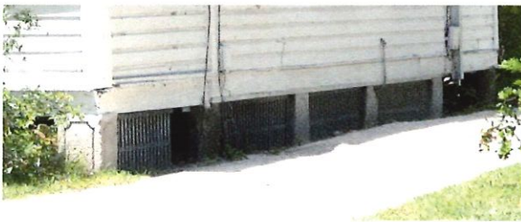
Coquina concrete block is a material unique to St. Augustine
