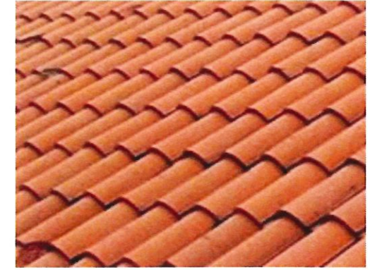
Clay tile roof
