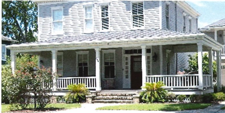
Wrap-around porch with columns and balusters, and front entry porch with columns and steps symmetrically aligned with front door
