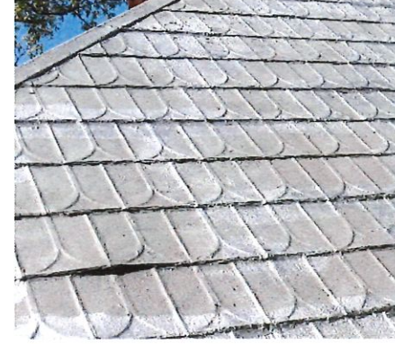
Stamped metal shingle roof
