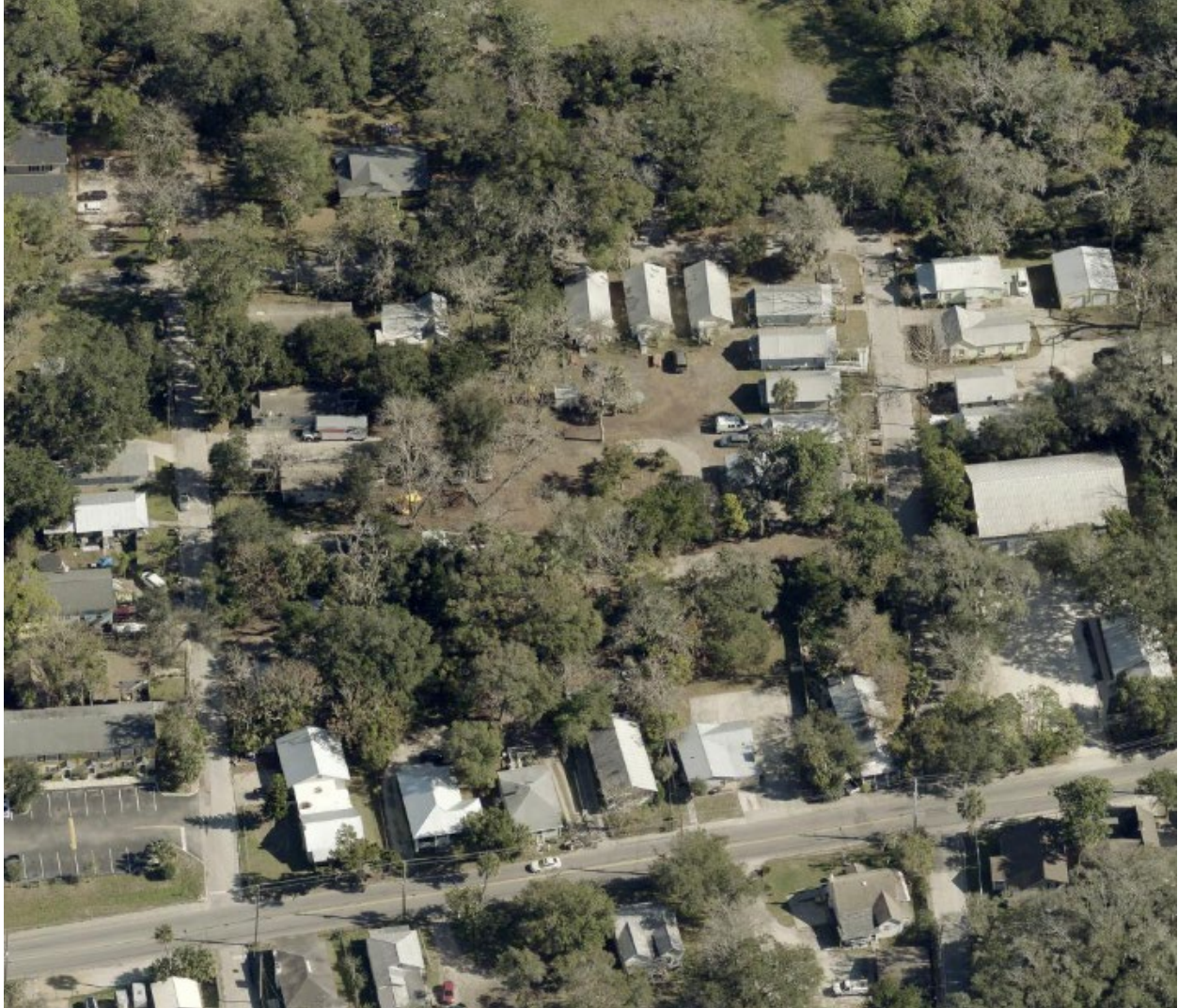
Figure 1. This aerial photograph shows the Emergency Services and Homeless Coalition Campus located in West City of St. Augustine.
