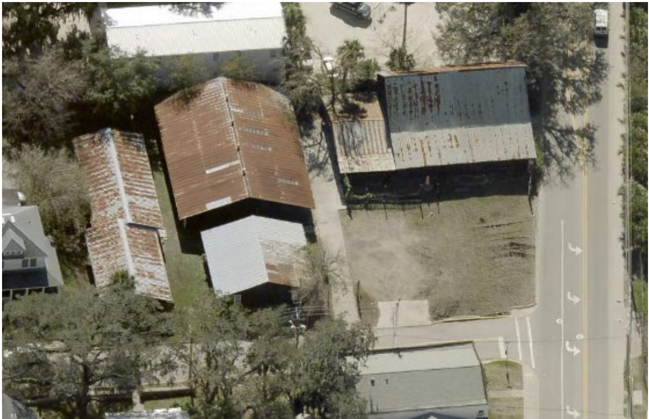
Figure 1. This photograph shows an aerial view of 115 La Quinta Place as it exists today.
