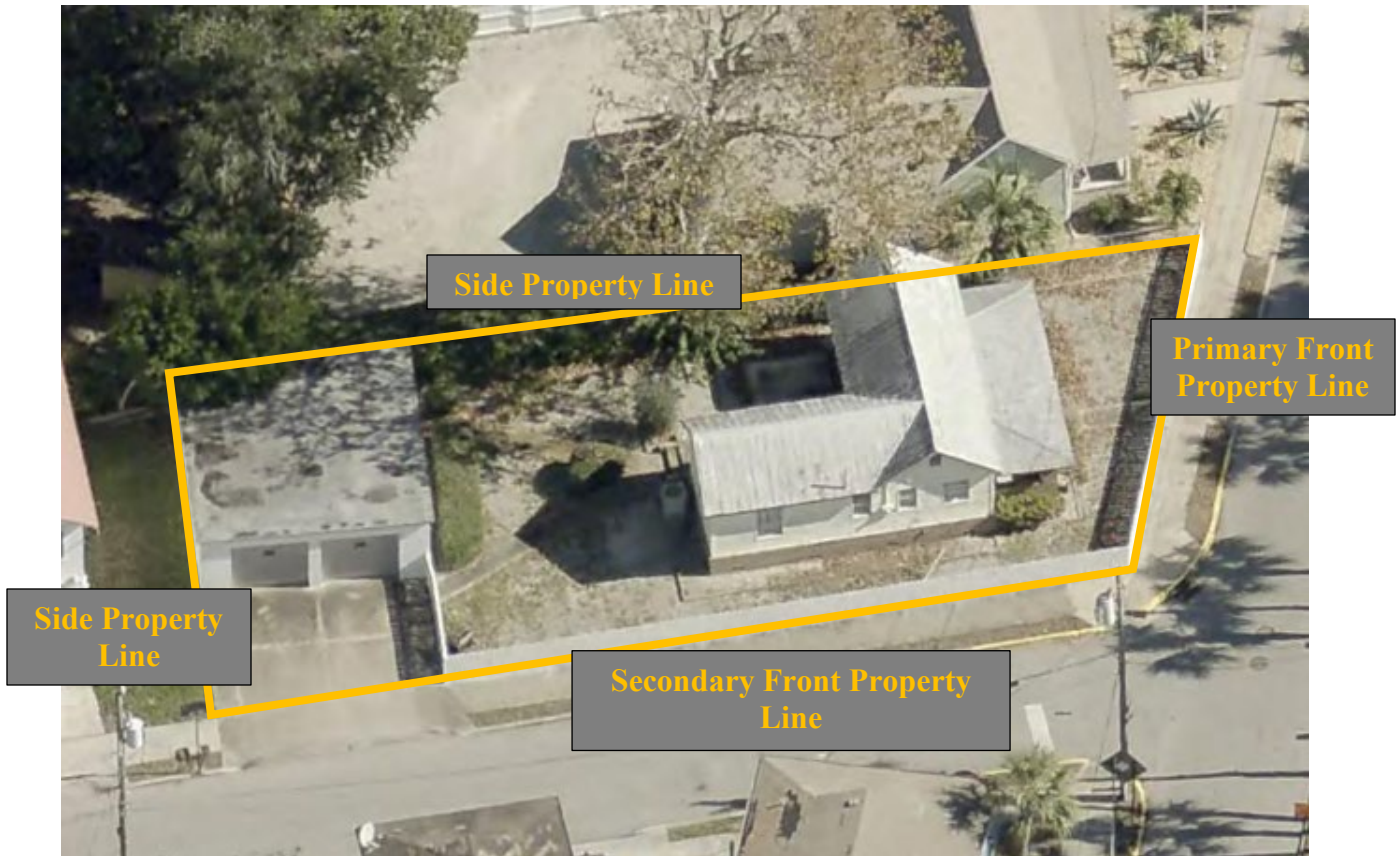
Figure 1. This aerial photograph shows the property at 8 Perpall Street. Located on the left side of the photograph is the existing garage where the proposed second floor addition is to take place.
