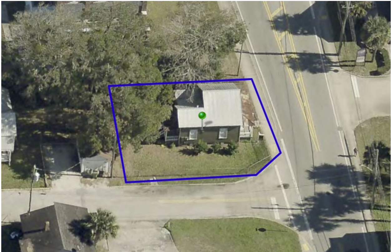
Figure 1. This photograph obtained through EagleView's CONNECTExplorer shows an aerial view of 260 W King Street.
