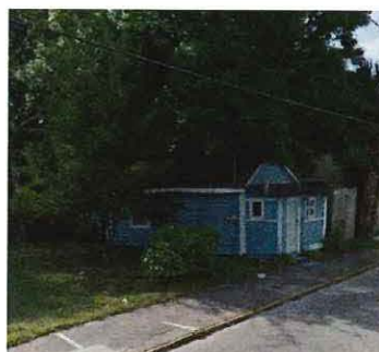
124 MARTIN LUTHER KING AVENUE | Frame Vernacular
