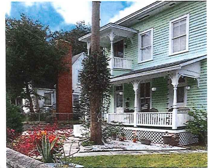
Piers with latticework. Image by ML+H.
