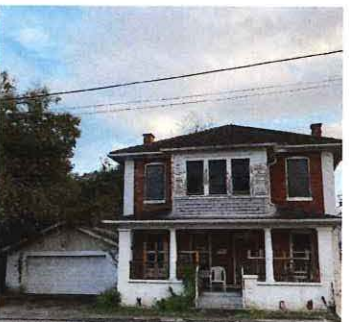
81 ST FRANCIS STREET | Masonry Vernacular
