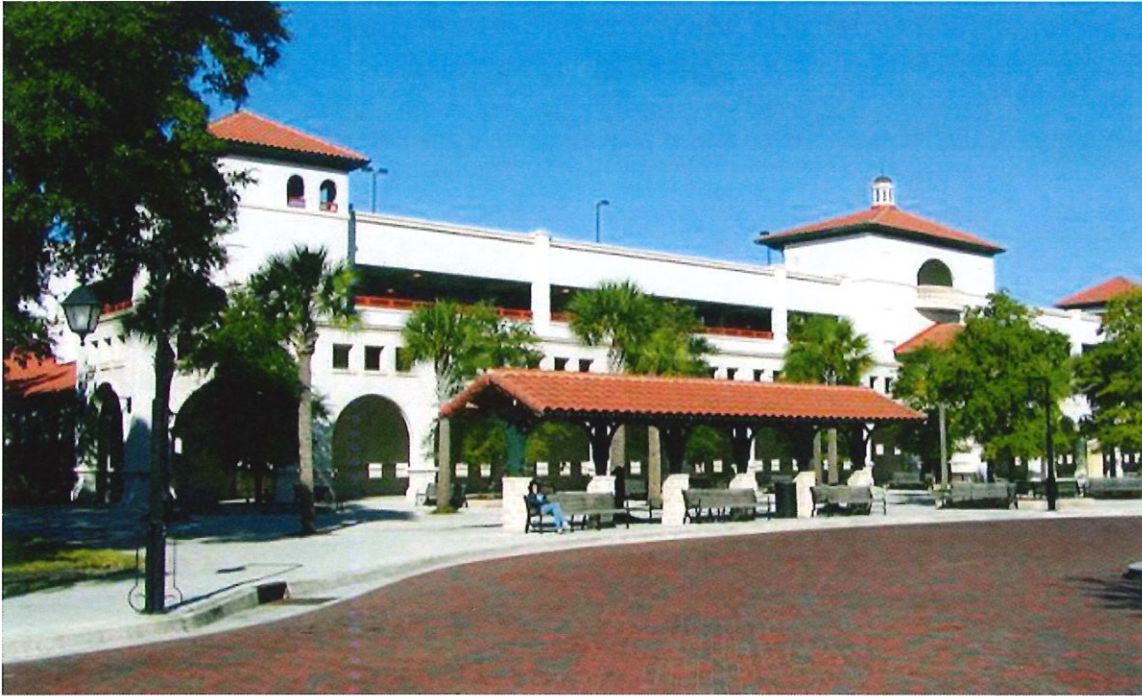
Figure 11. Historic Downtown Parking Facility (Garage)
