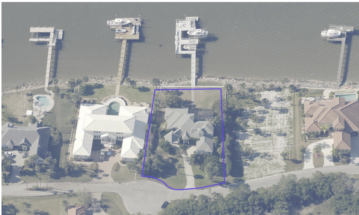
Figure 1. Aerial photograph of the subject property.
