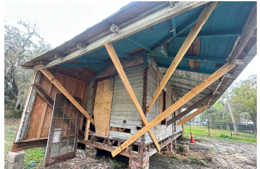
Previously enclosed Northwest corner (door to become window)
