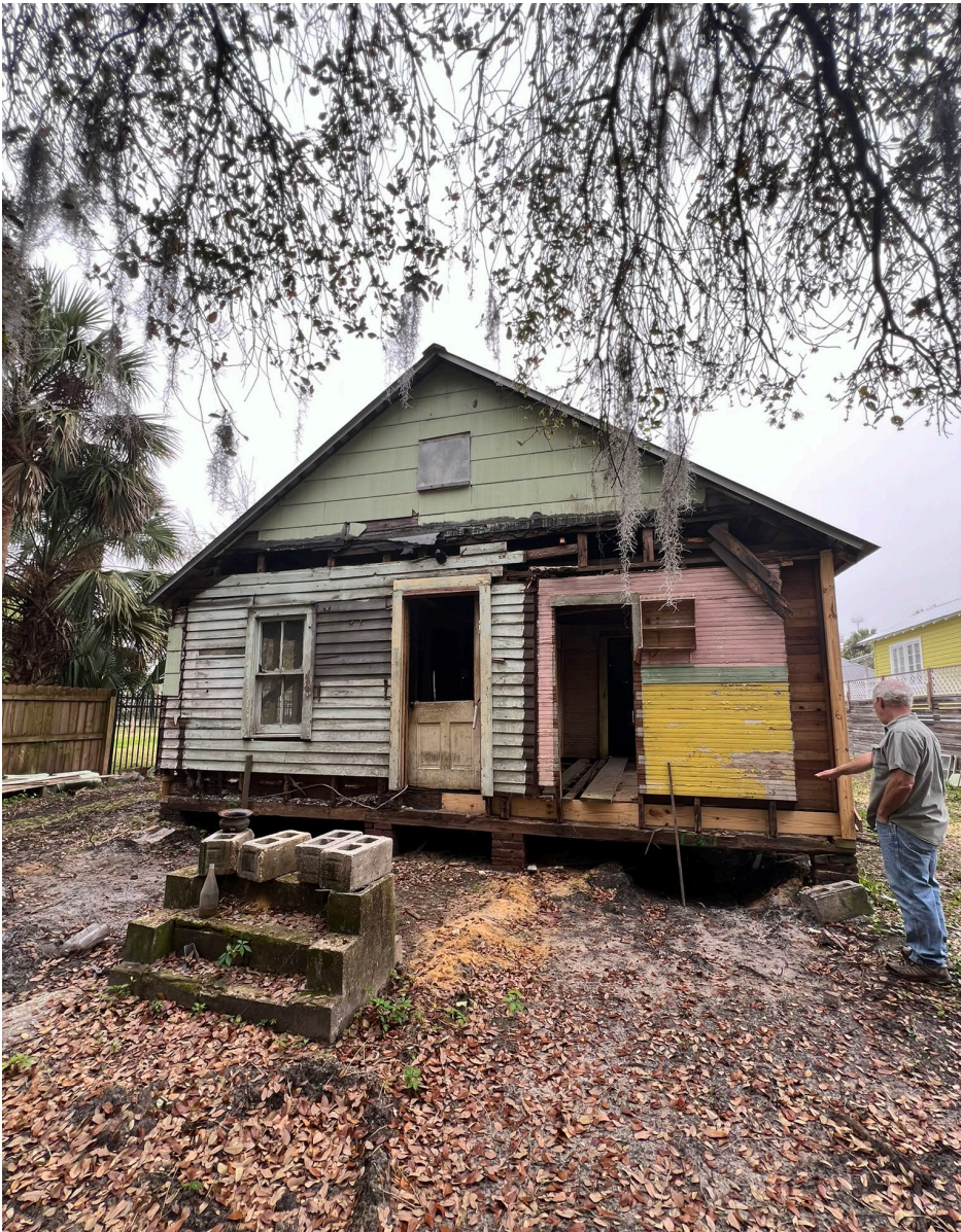
Rear elevation, location of previously existing enclosed porch (note concrete steps)
