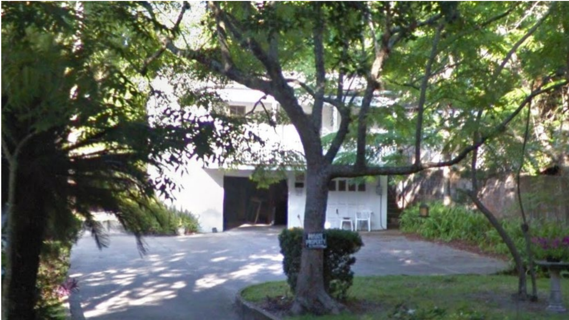
2013 Google Streetview of Cantilevered Porch
