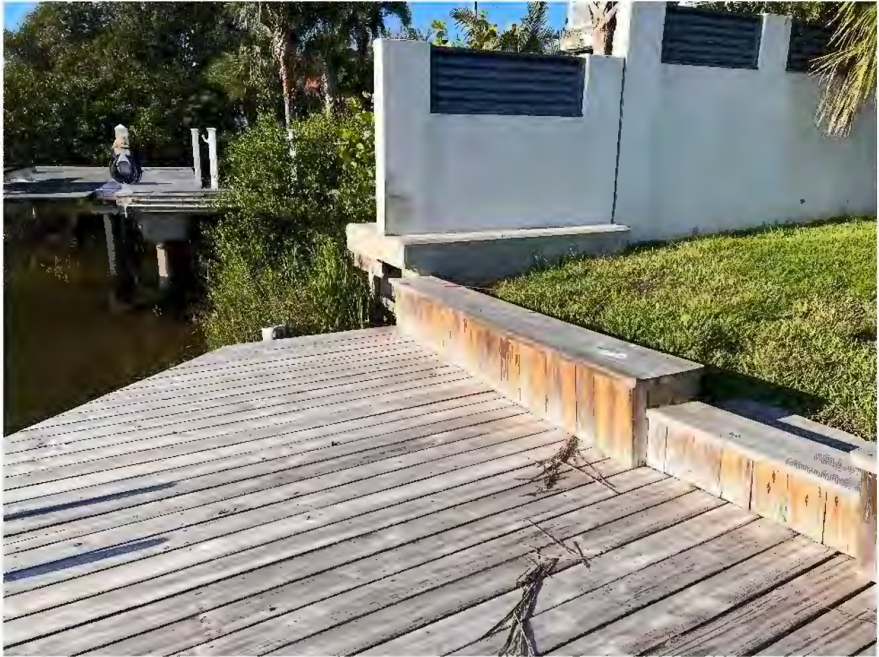
Neighbor to the south bulkhead and section of existing bulkhead
