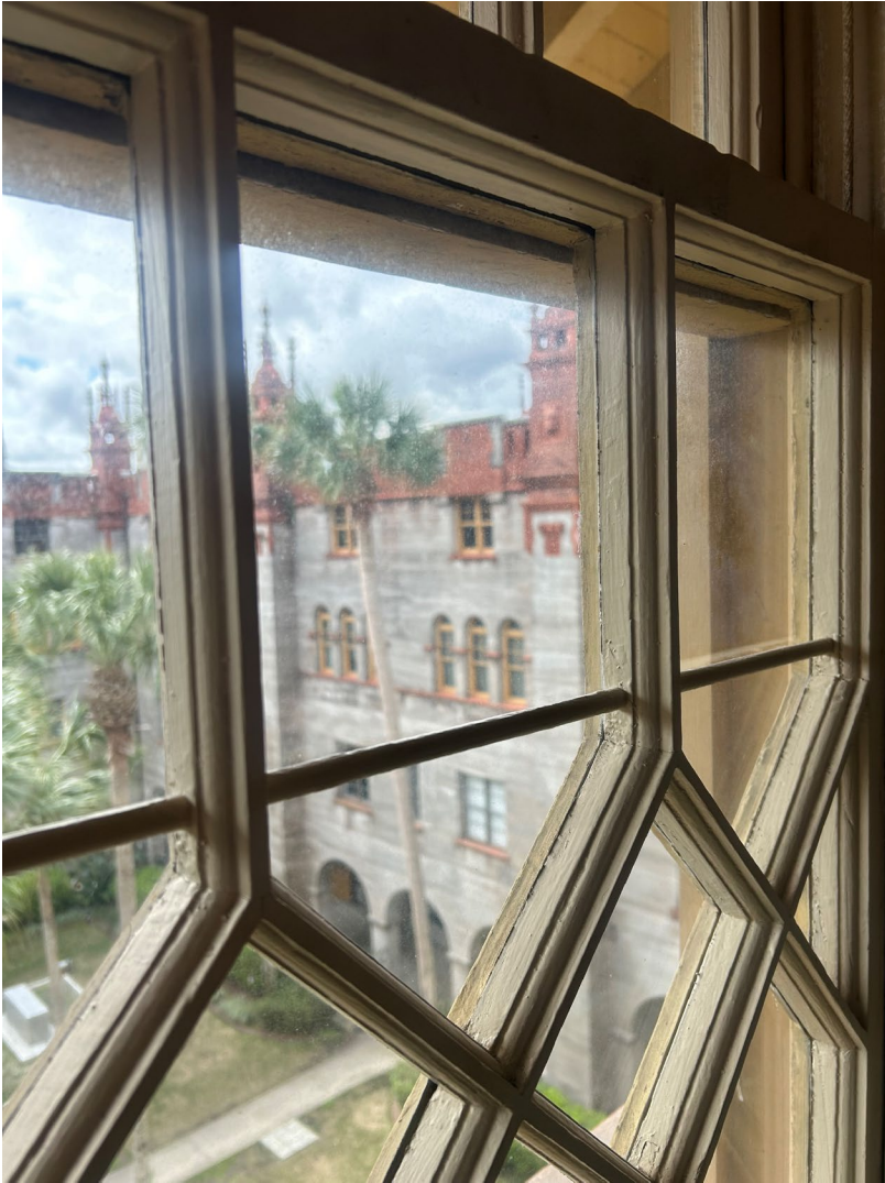
North Elevation, 4 th Floor: Historic wood windows with double hung sashes, sash cords in place, and what is said to be documented historic color
