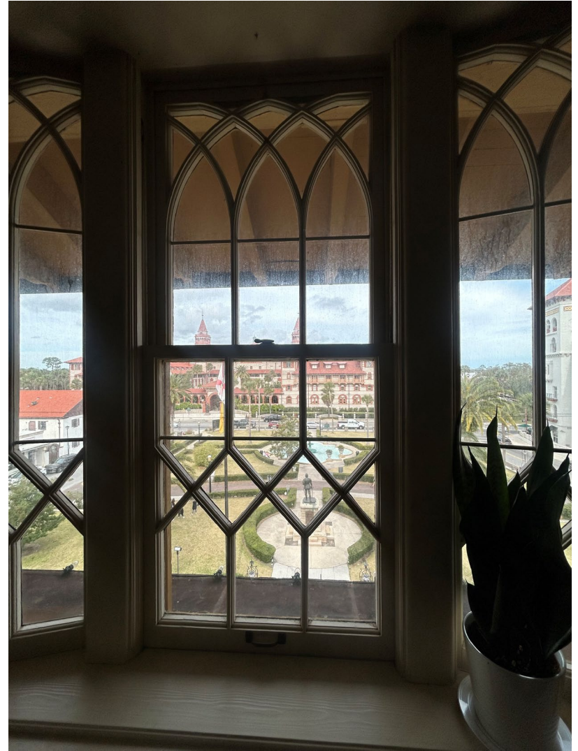
North Elevation, 4 th Floor: Historic wood windows with double hung sashes, sash cords in place, and what is said to be documented historic color
