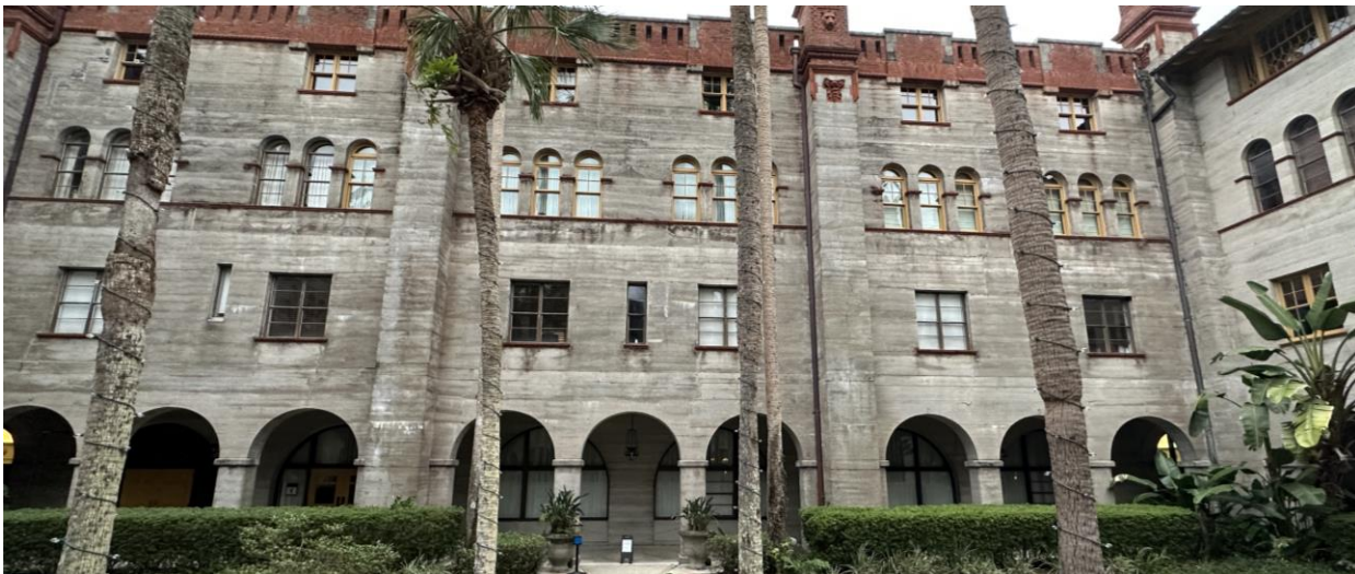
Existing and replacement windows
