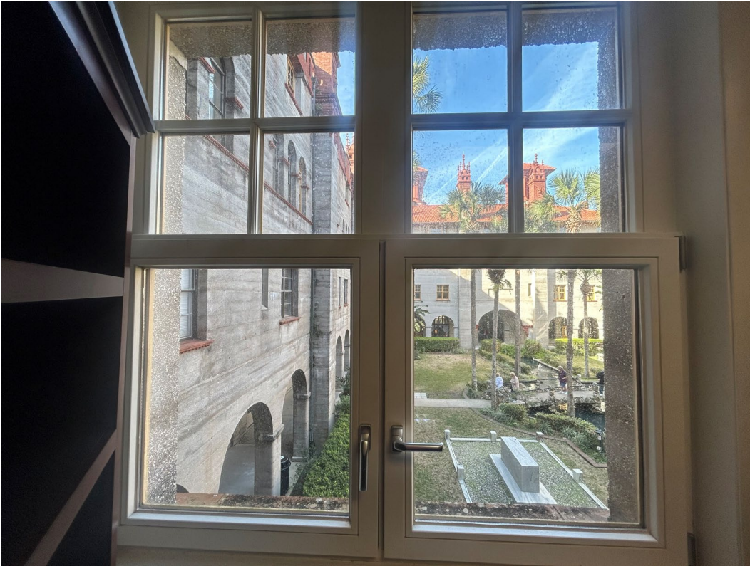
Interior view of windows on 2nd Floor (above Lightner Museum entrance): Rema wood windows approved by the HARB in 2000
