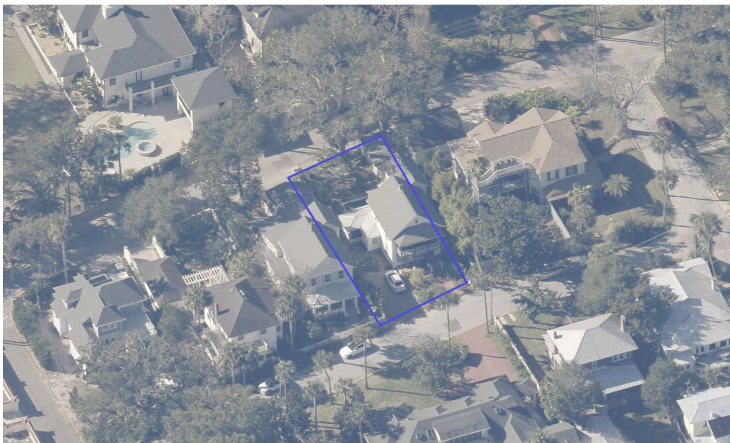
Figure 1. Aerial photograph of the subject property.
