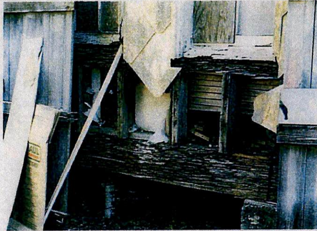
Image 5: Exposed Floor Beam and Wood Studs
