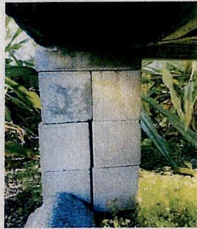
Image 2: Hollow Block Stacked Pier
