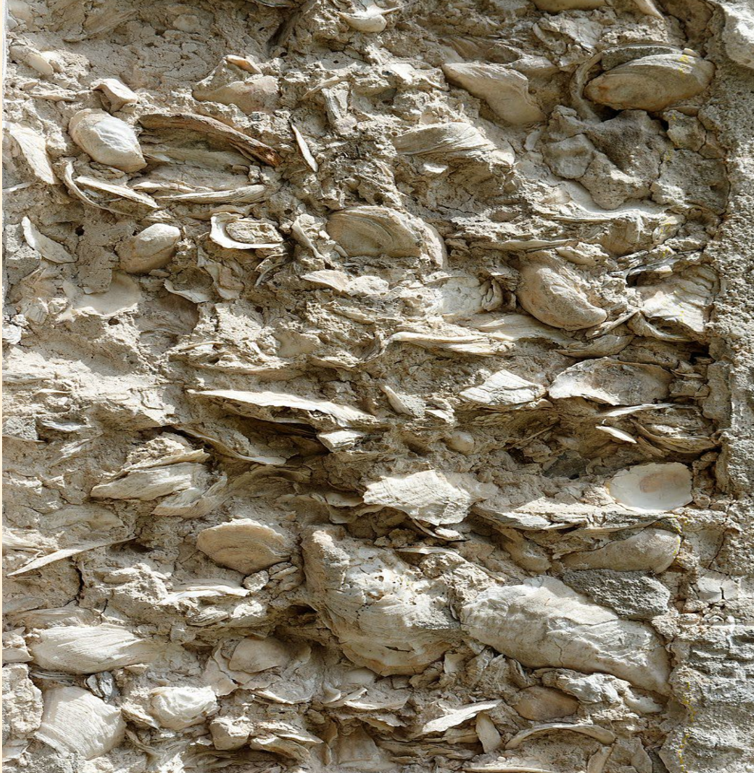
FIGURE 18 TABBY STRUCTURAL WALL
