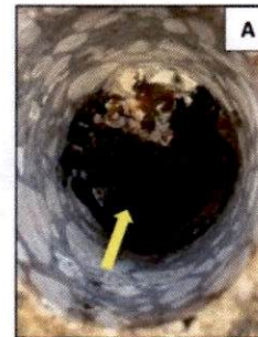
Figure 1: Crack inspection, drilling cores, and rebar inspection. A) Evident corrosion product at the bottom of the core; B) Core extraction; and C) Delamination at the level of the steel rebar.
