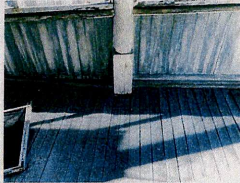
Image 10: Sloped Decking
