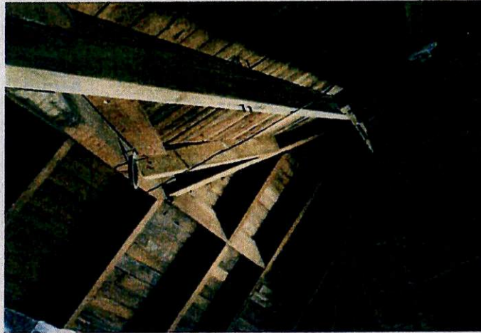
Image 11: High Roof Framing from Attic Access
