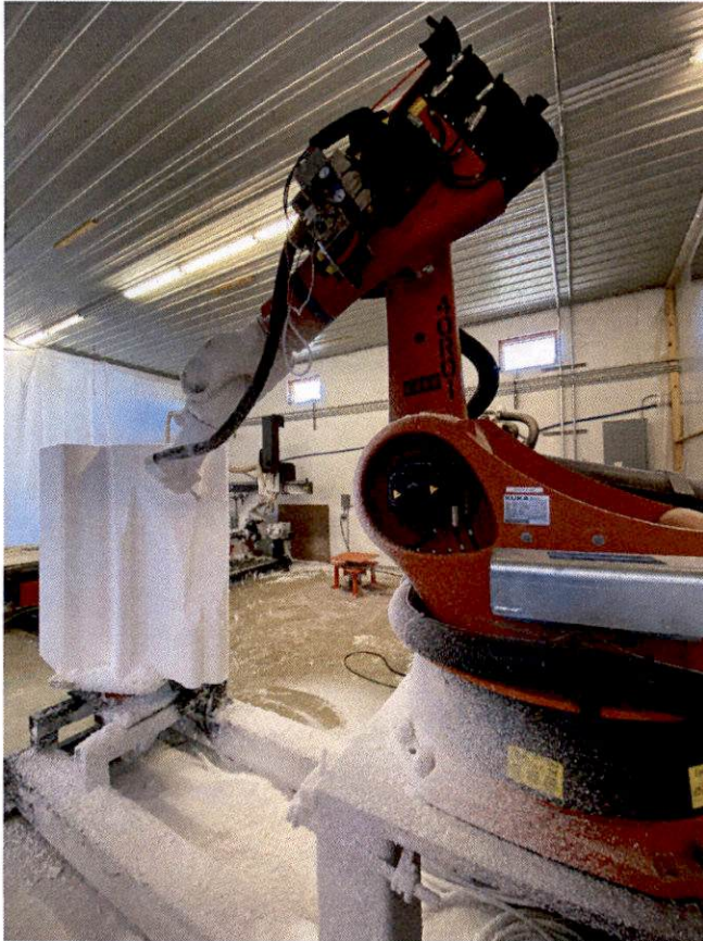
CNC Routed Foam Used for Formwork
