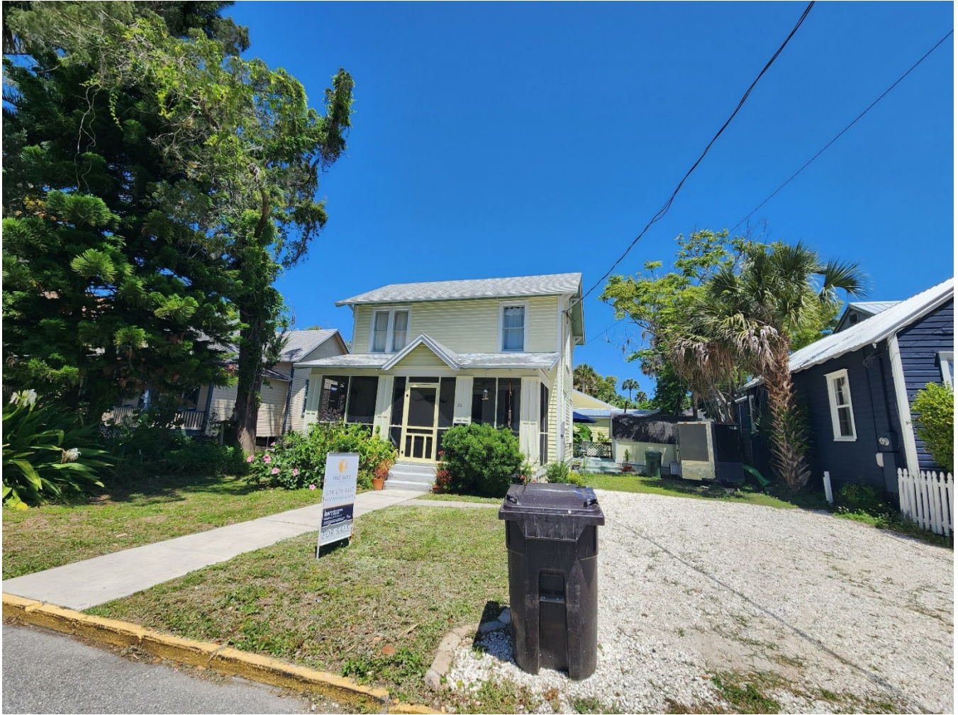
Photo 9. 26 Joiner Street, facing north. Meghan Browning, photographer; April 29, 2024.
