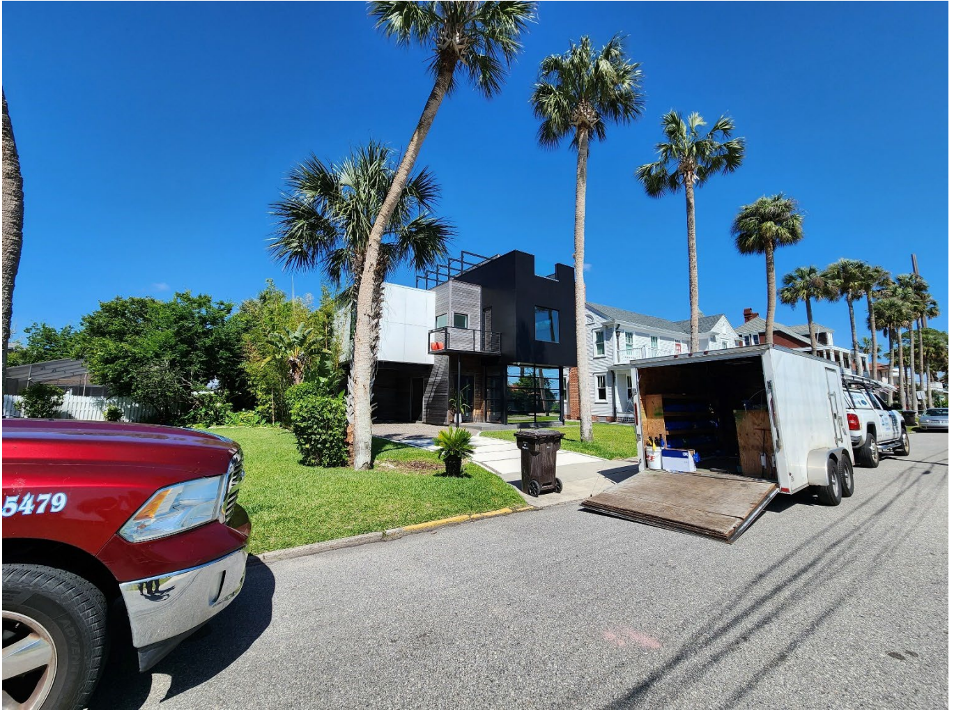
Photo 18. Water Street, facing northwest. 68 Water Street (2007) is the geometric building to the far left (south). Meghan Browning, photographer; April 29, 2024.
