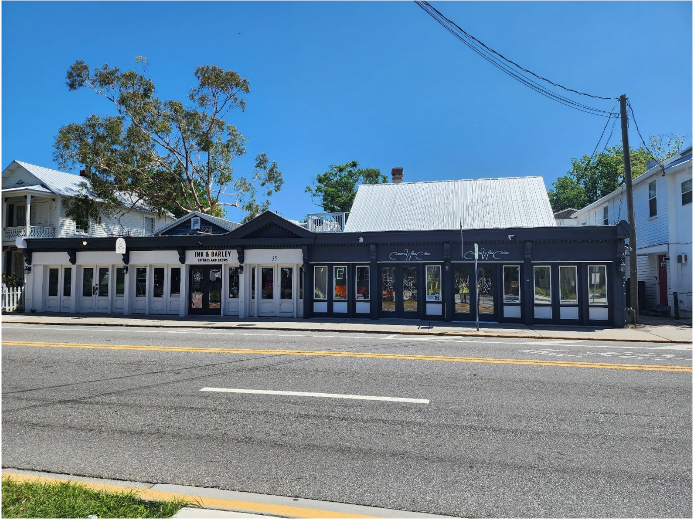
Photo 5. 35 San Marco Avenue, facing southeast, with 31 San Marco Avenue partially visible behind it (to the south). Meghan Browning, photographer; April 29, 2024.
