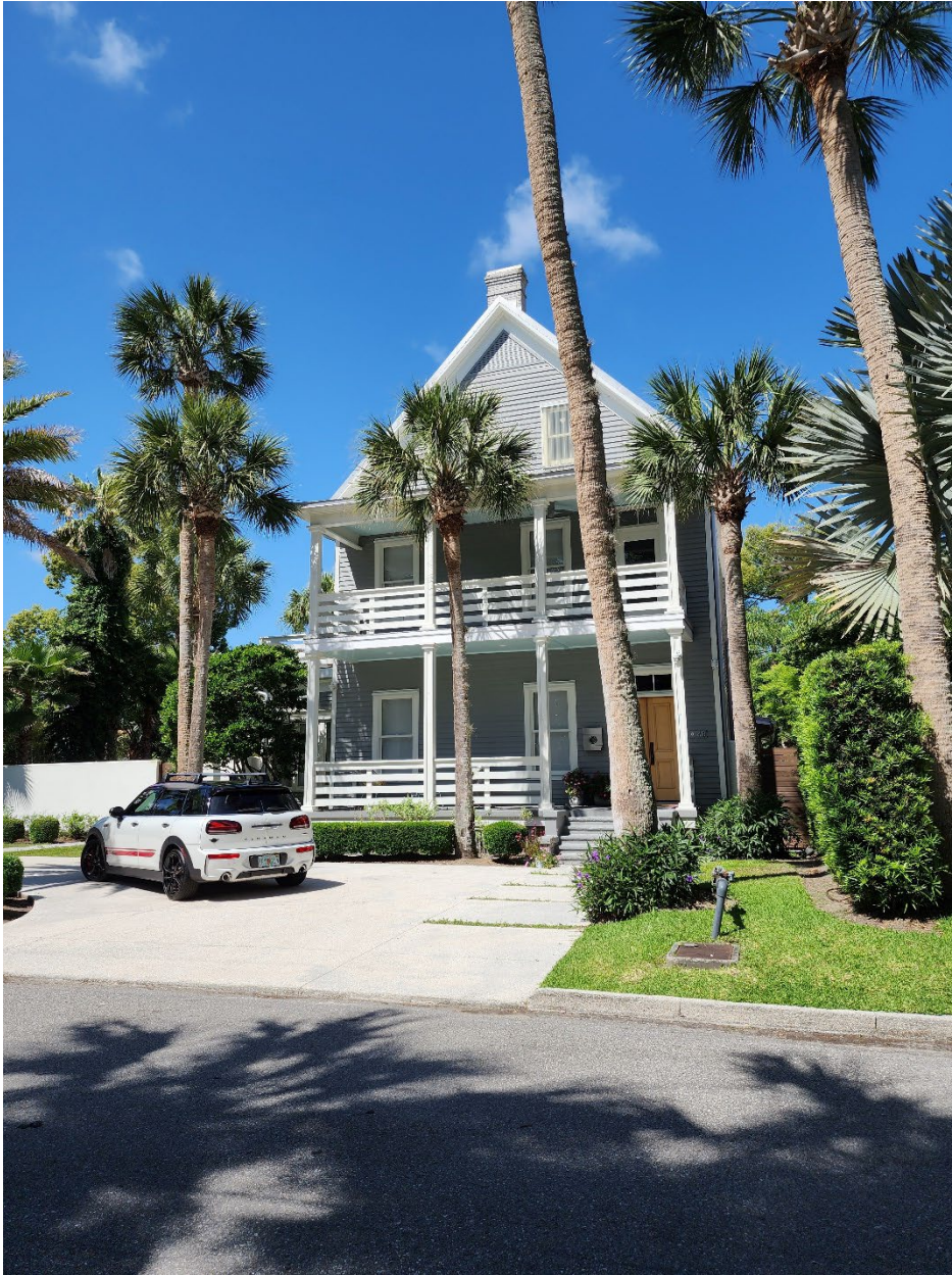
Photo 5. The Abbott House at 48 Water Street, facing west. Meghan Browning, photographer; April 29, 2024.
