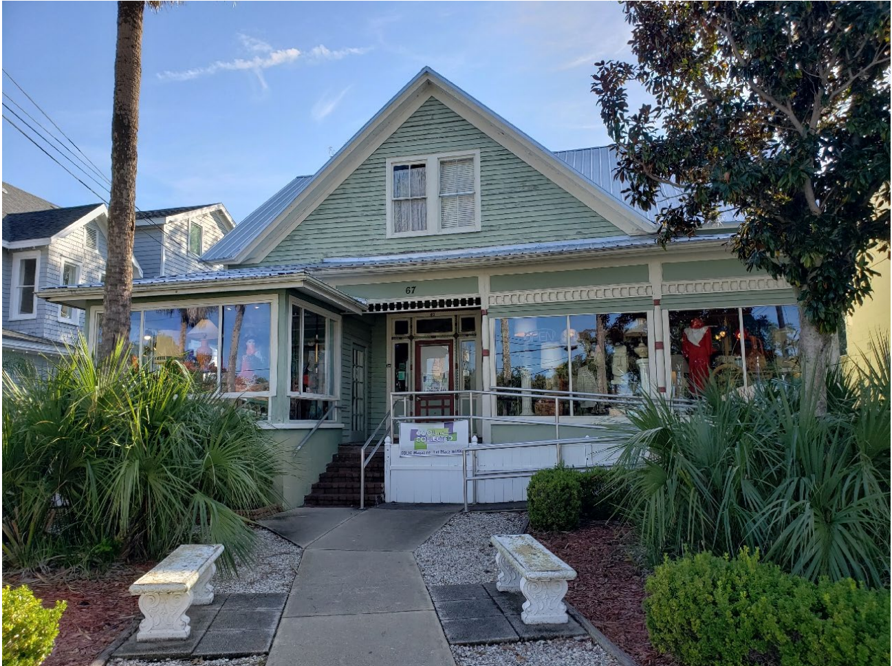
Photo 8. 67 San Marco Avenue, facing east. Katie Fitzpatrick, photographer; October 2, 2020.
