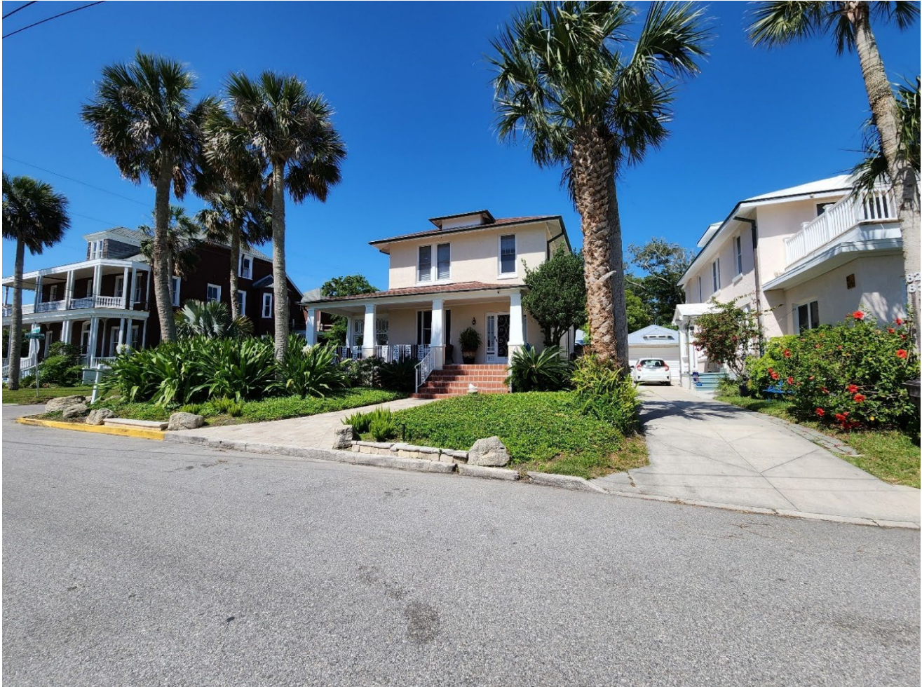
Photo 1. 82 Water Street, facing northwest. Meghan Browning, photographer; April 29, 2024.
