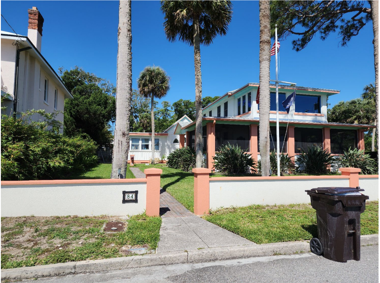
Photo 3. 84 Water Street, facing northwest. Meghan Browning, photographer; April 29, 2024.
