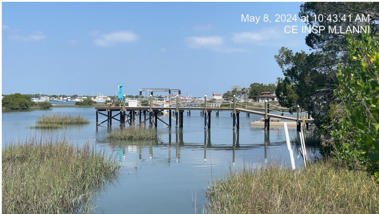
Image of boatlift - 81 Coquina Ave.
