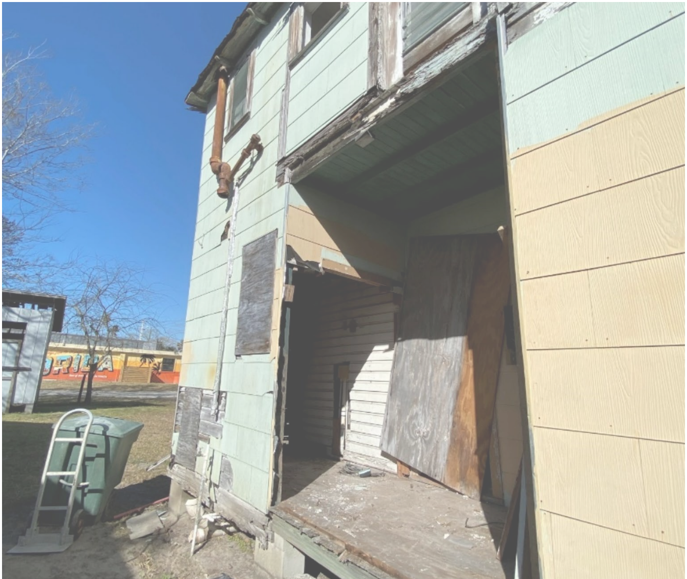
Figure 2. Photograph from February of 2022 showing the previous shed, seen in the far left of the picture, at 148 Cunningham Avenue.
