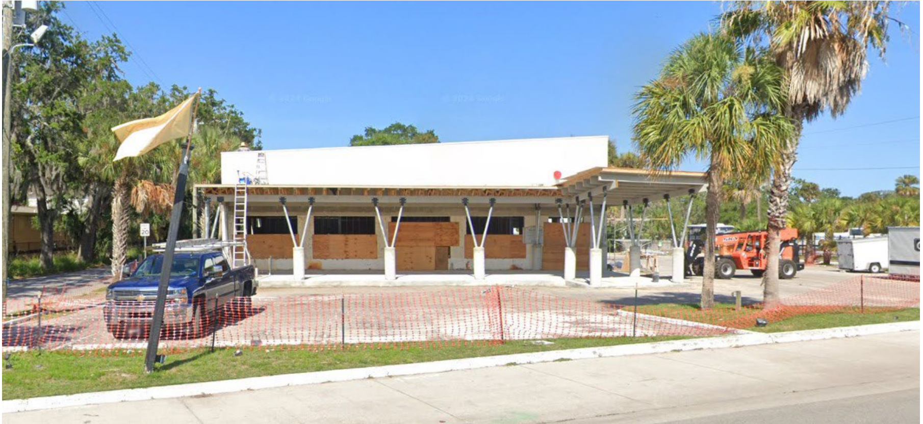
Front (west) Elevation – May 2024 Google Street View
