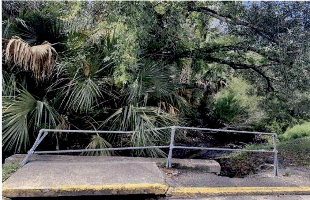
VIEW OF THE DRAINAGE DITCH RUNNING THROUGH THE SUBJECT SITE
