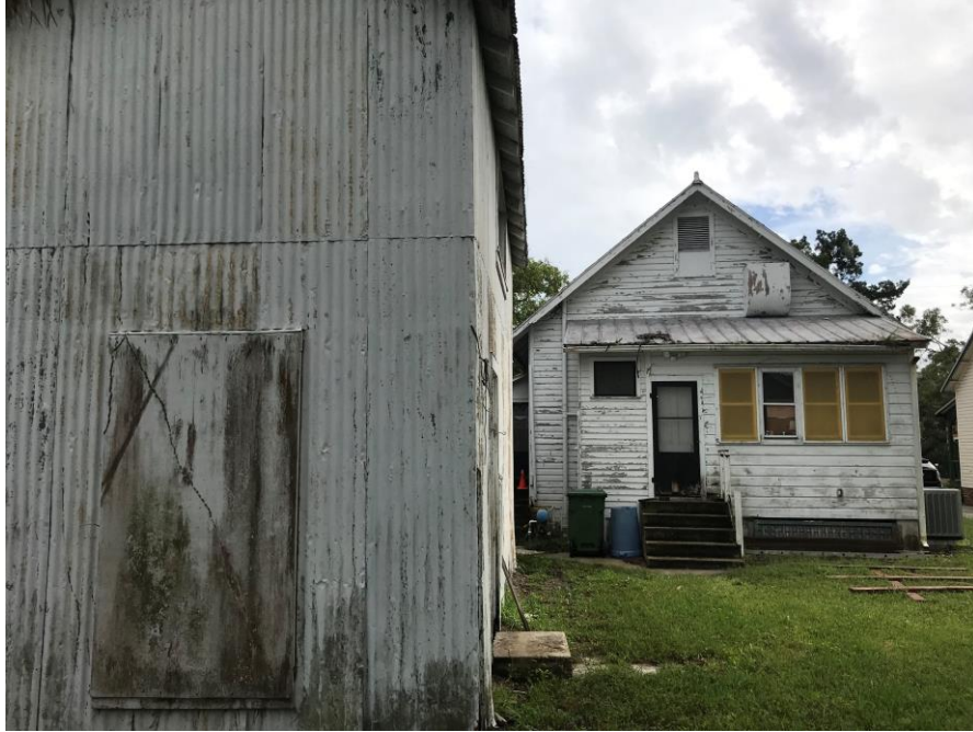
Facing south at back of property
