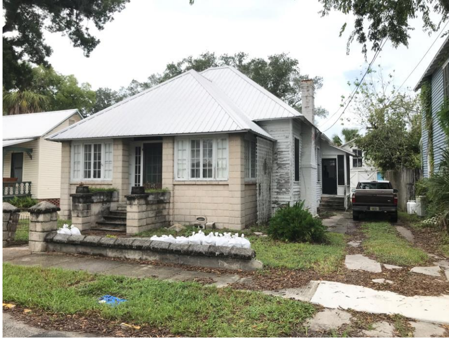
22 Grove Avenue primary structure
