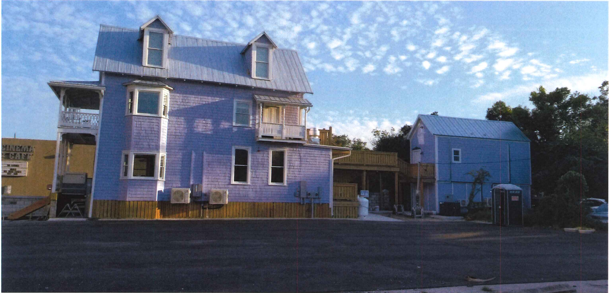
Photo 4 Primary and Auxiliary Structures North Side Façade, View South from City Parking Lot Photographer: Leslee Keys, September 17, 2019
