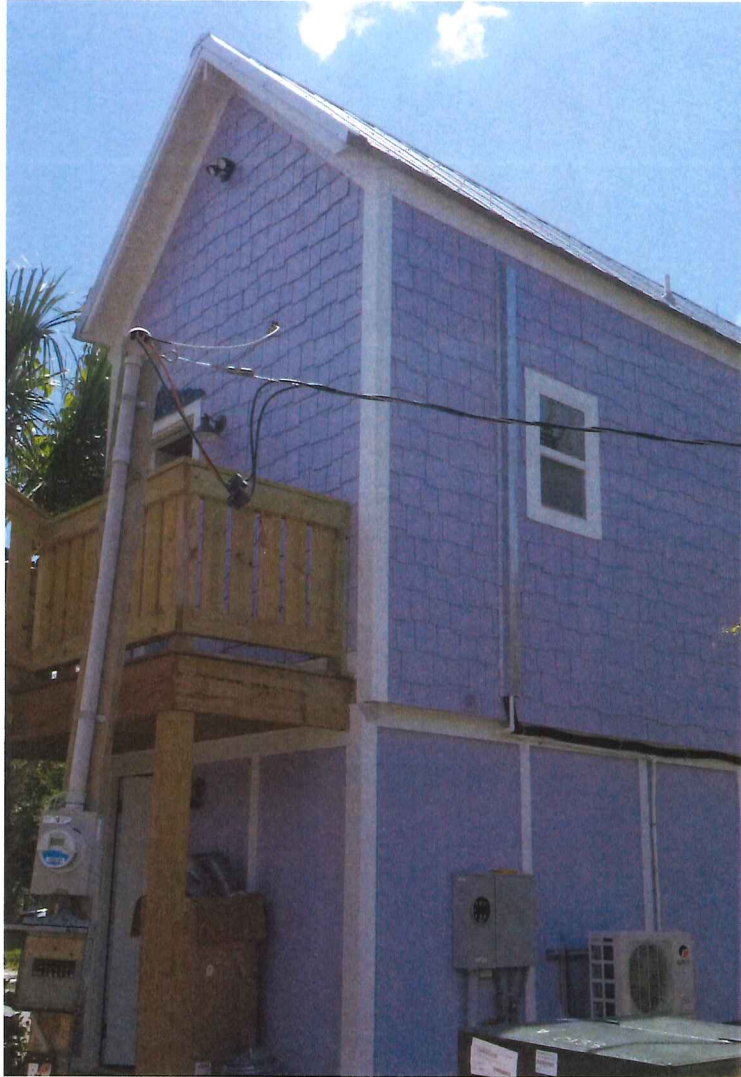
Photo 10 East - Front Façade, View West from parking lot Photographer: Leslee Keys, September 16, 2019
