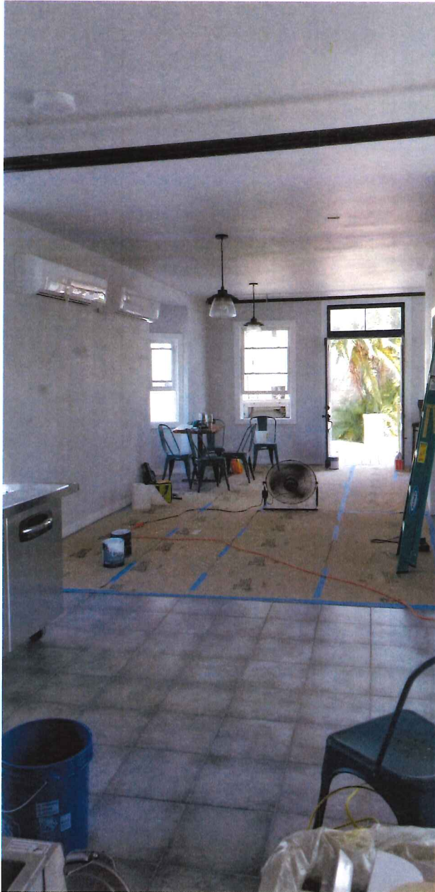
Primary Structure - Interior
