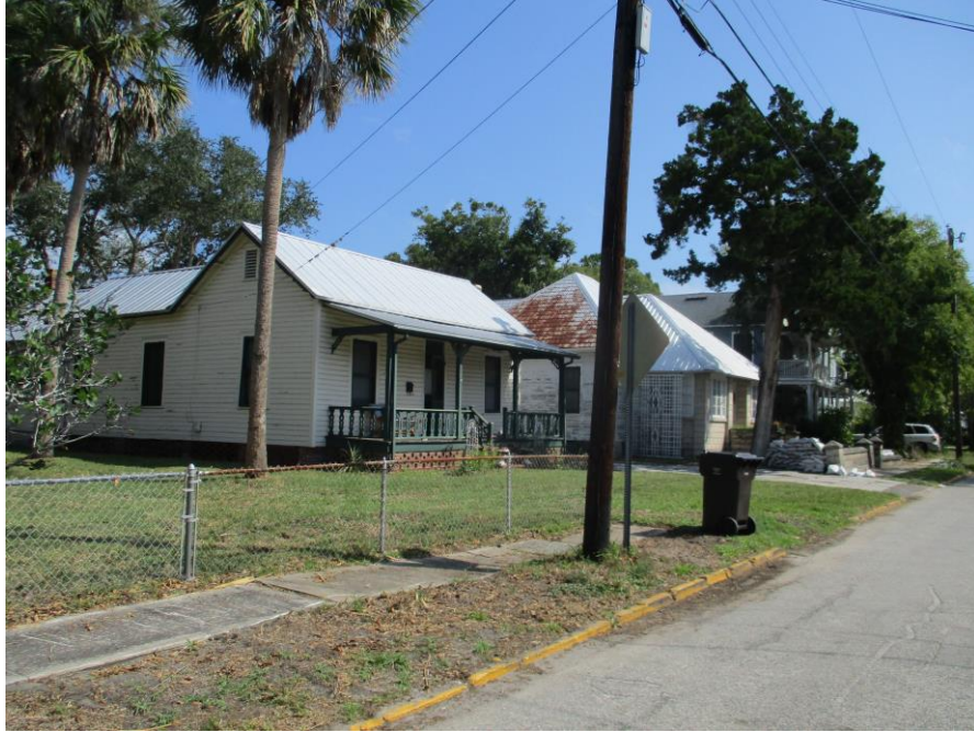
Context area facing northeast, subject property in the center
