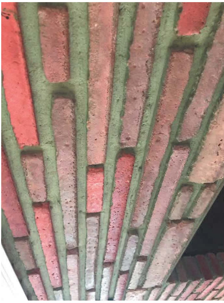
Detail of concrete brick fireplace
