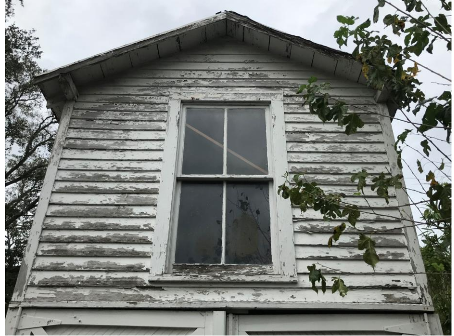
South elevation, second floor window
