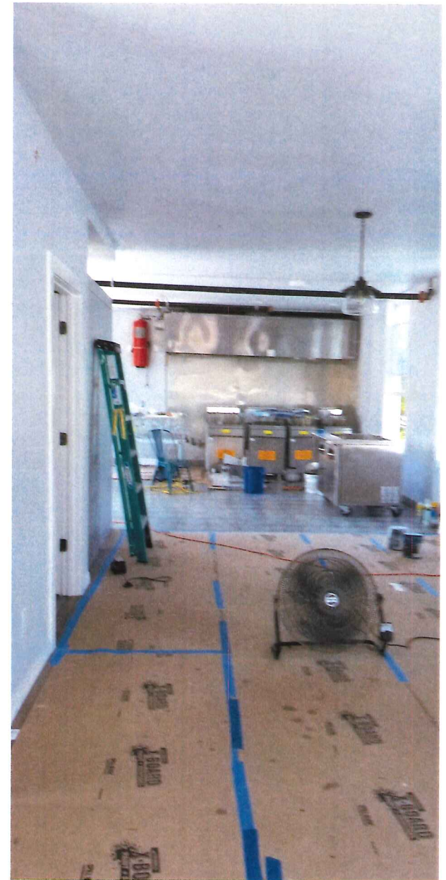
Photo: 7 First Floor West – Kitchen from Dining Area
