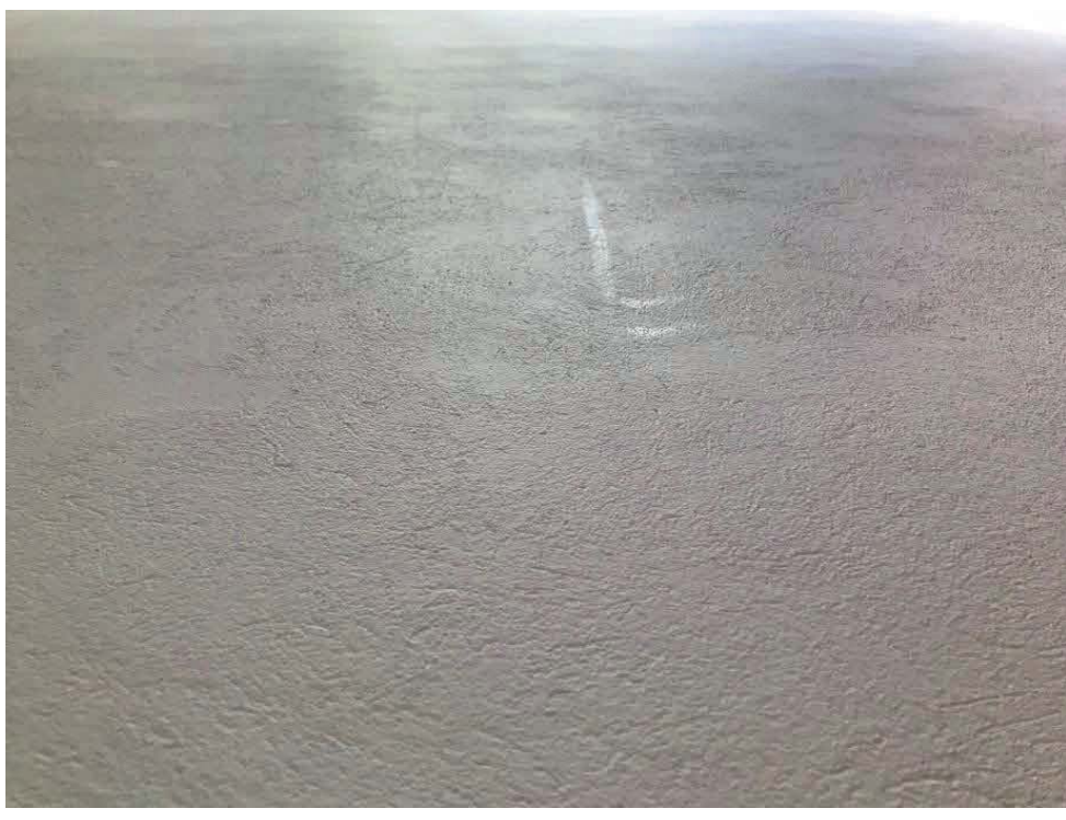
Plaster finish of walls
