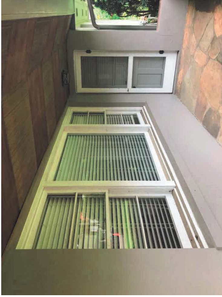
Front porch, secondary entry
