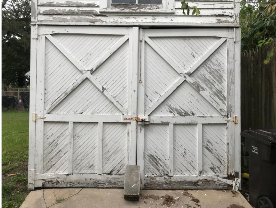
South elevation, first floor doors
