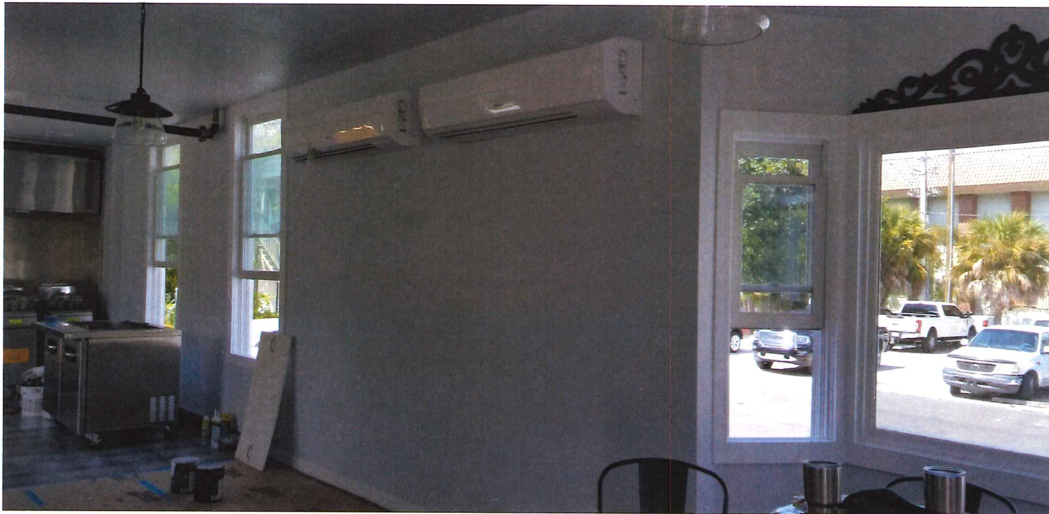
Photo 8 Primary Structure – Interior First Floor View W/NW – Dining Area Photographer: Leslee Keys, September 16, 2019
