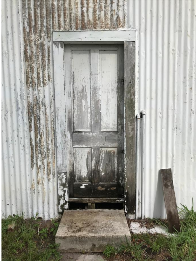
West elevation door
