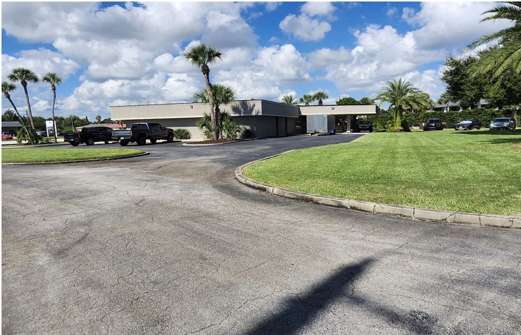
REAR AND SIDE VIEW OF THE SUBJECT BUILDING LOOKING WEST
