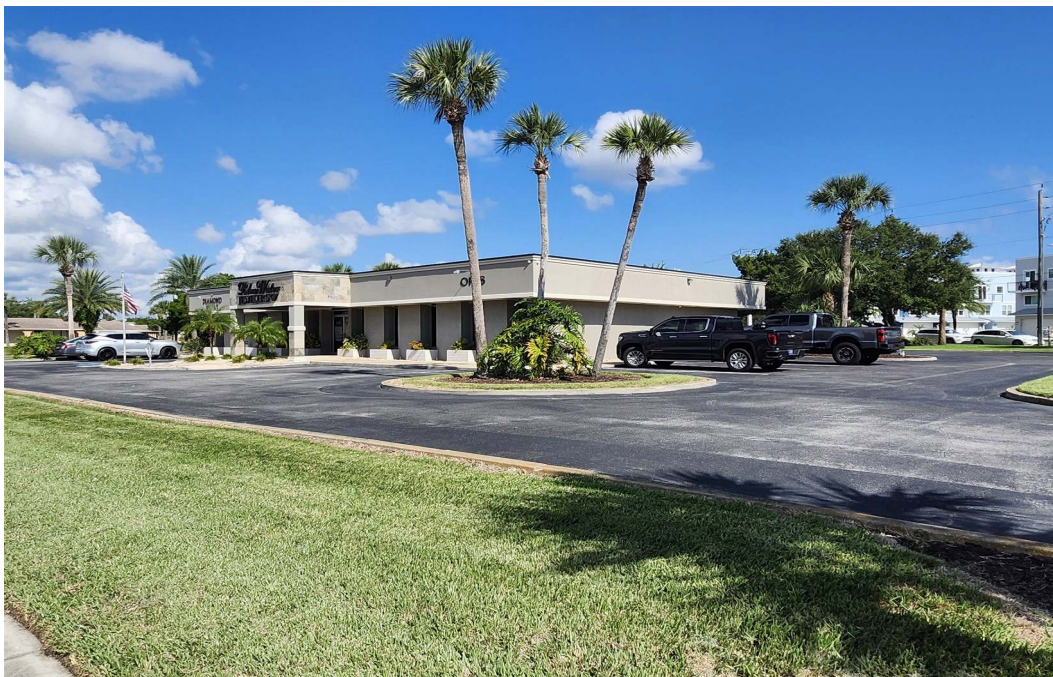
FRONT VIEW OF THE SUBJECT LOOKING NORTHWEST FROM ANASTASIA BLVD.
