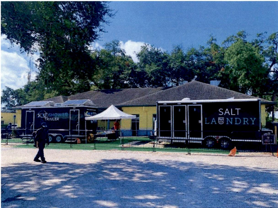
SALT Exterior Facilities | Orlando, FL
