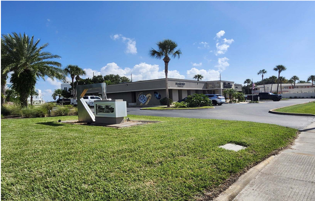
FRONT VIEW OF THE SUBJECT LOOKING NORTHEAST FROM ANASTASIA BLVD.
