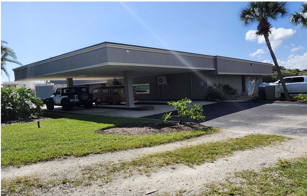
REAR AND SIDE VIEW OF THE SUBJECT BUILDING LOOKING SOUTH
