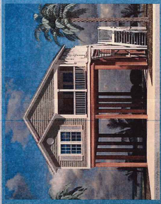
Elevation By Columns/Piers/Slab
