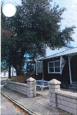
Masonry site walls with floodgates can provide flood protection. Image from ML+H.
