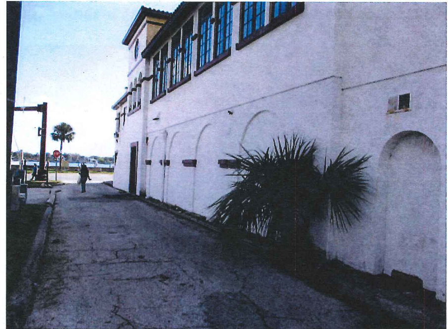
North elevation near the rear of the building, arched loggia to be opened
