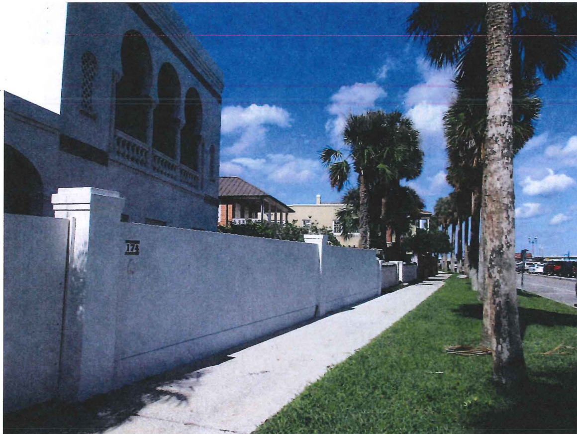
174 Avenida Menendez wall, looking north towards 168 Avenida Menendez
