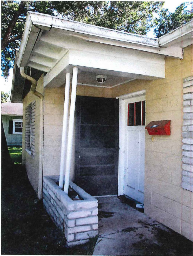
Front Entrance on North Elevation: facing southeast
