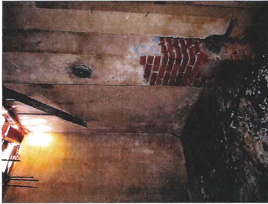
Interior with brick chimney, likely original exterior wall
