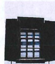
Window on the Front Elevation
