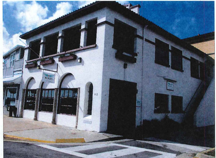
NE corner at Cuna Street, arched windows to be opened, stair removed, entry altered
