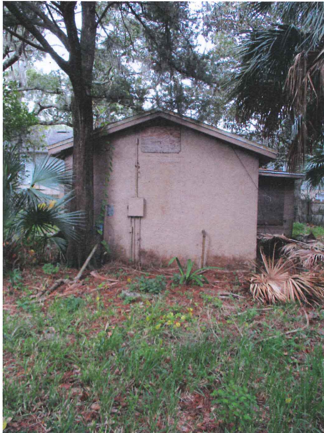
North Elevation: facing south
