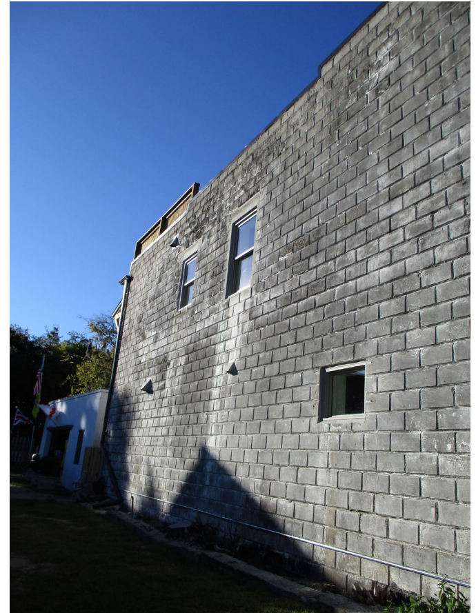
South Elevation: looking northwest
