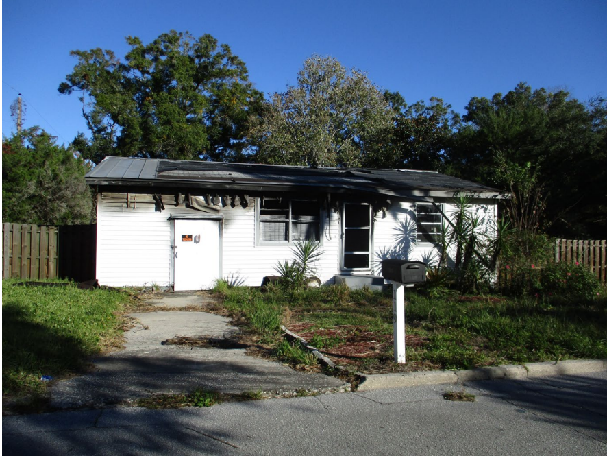
Front Façade / West Elevation: looking east
