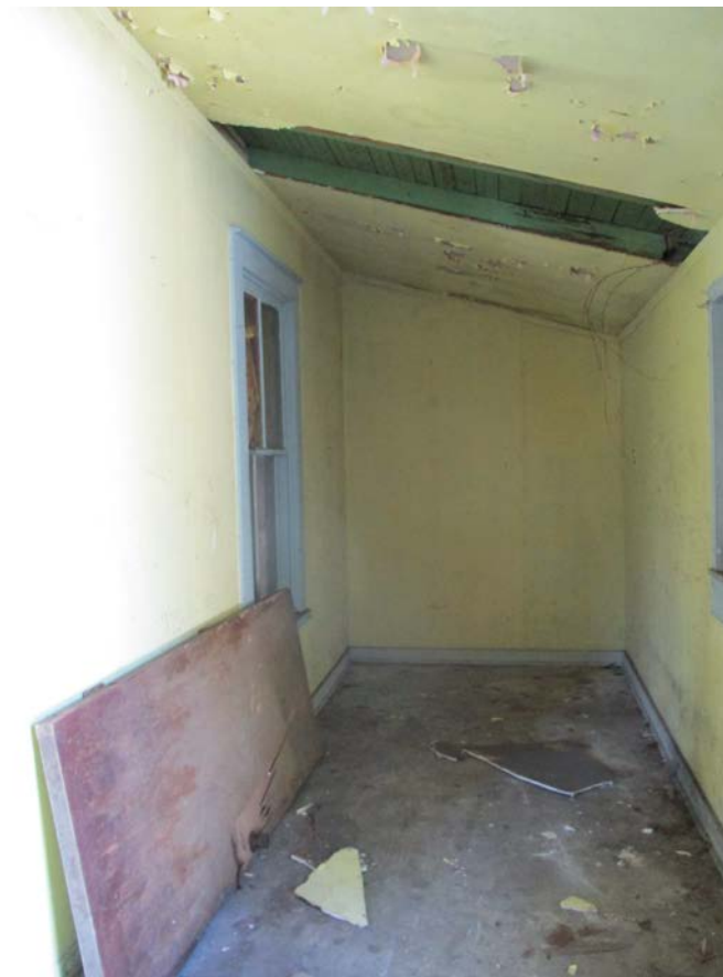
Enclosed front porch
