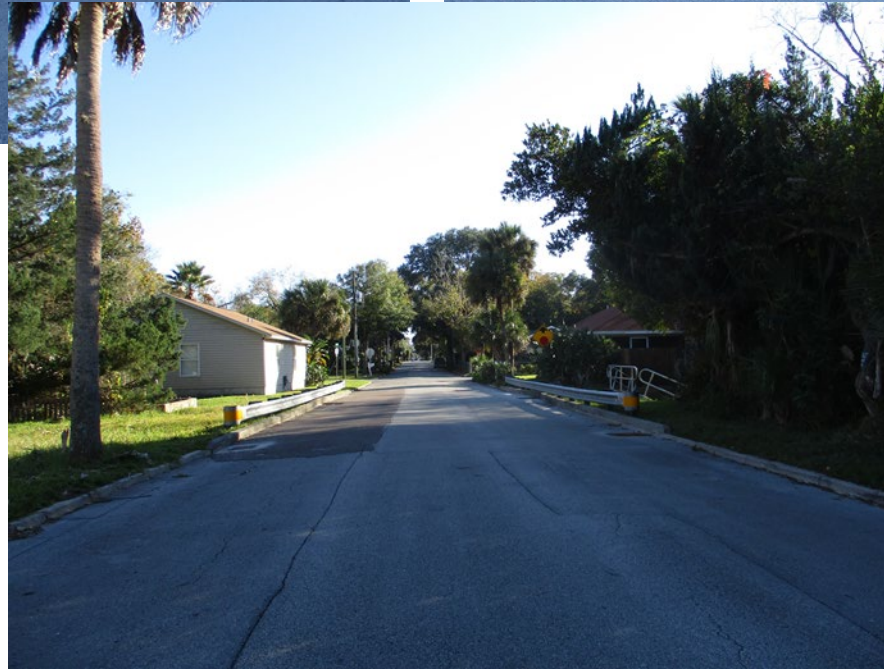
Looking south of the property
