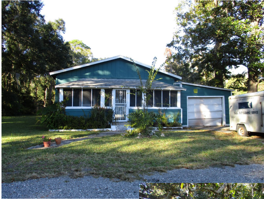
Front Façade / South Elevation: looking north
