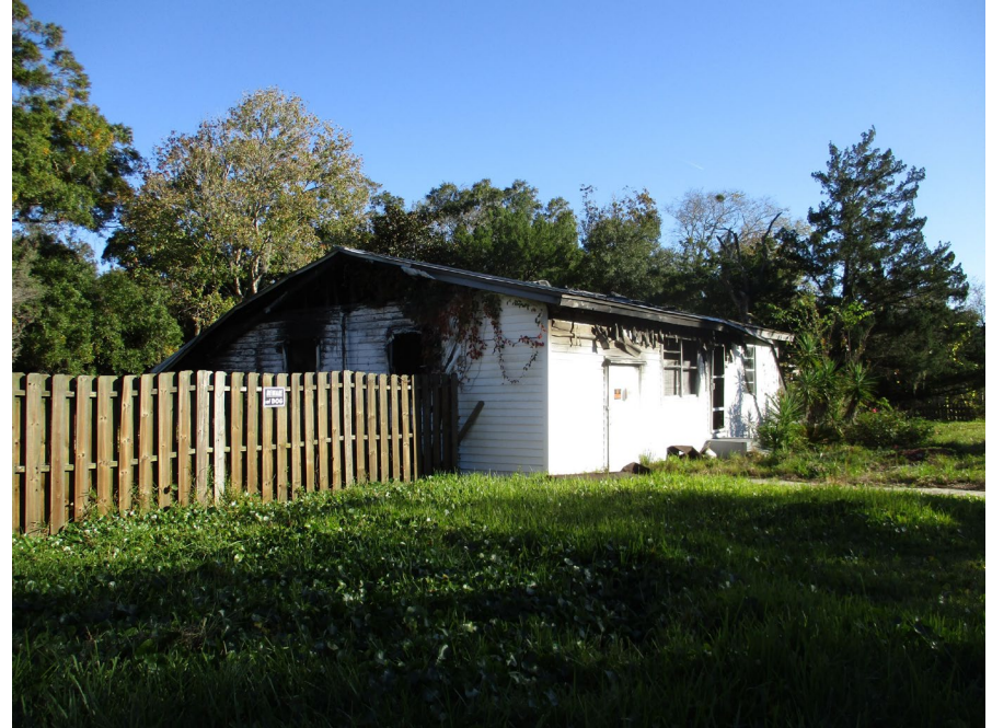
Northwest Elevations: looking south / southeast
