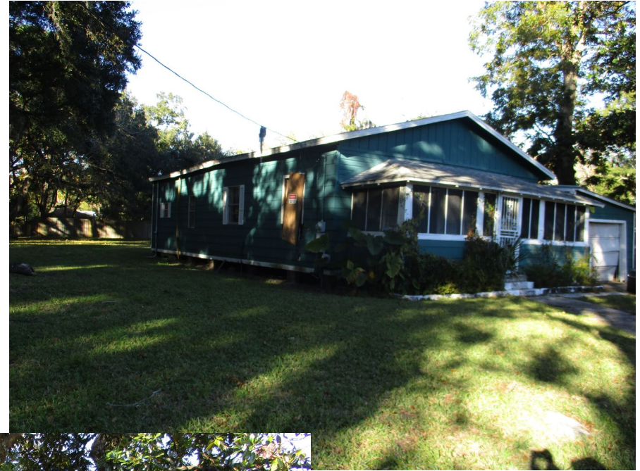
Southwest Elevations: looking northeast
