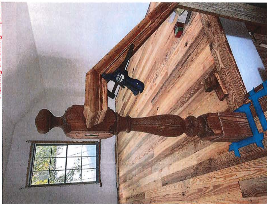
20240117121_KingsFerryWay_Staircase_002_1186 Notice how the additional height was derived from heart pine blocks at the base 86
