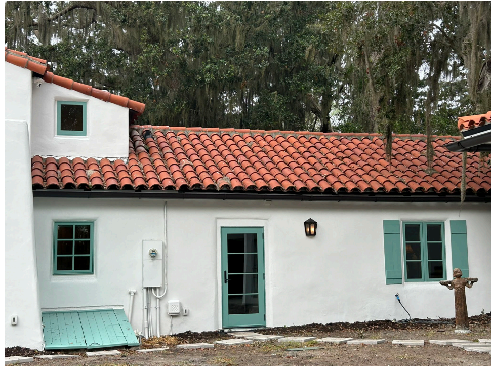
Existing Clay Tile on center two-story portion and north wing
