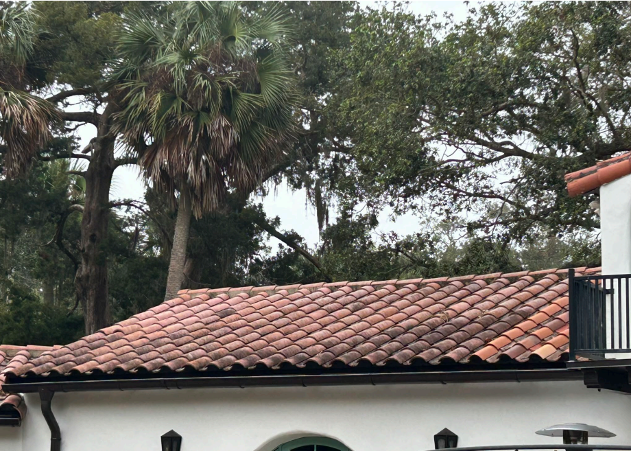
Existing Concrete Tile on south wing
