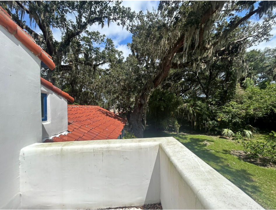
Roof deck on east elevation: accessed from 2 nd Floor
