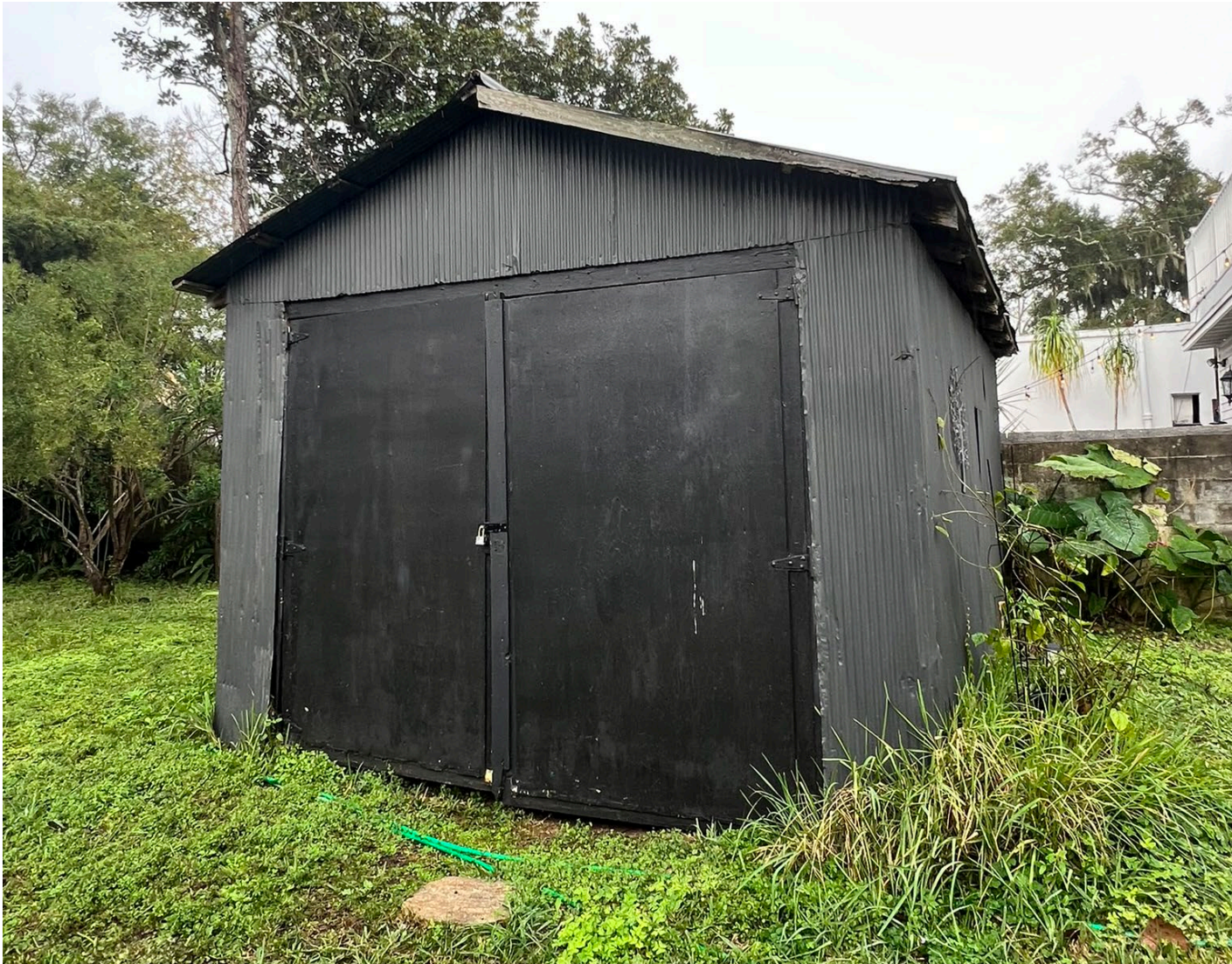
Shed proposed for demolition (noted on Sanborn Maps as 47-1/3 Abbott Street)
